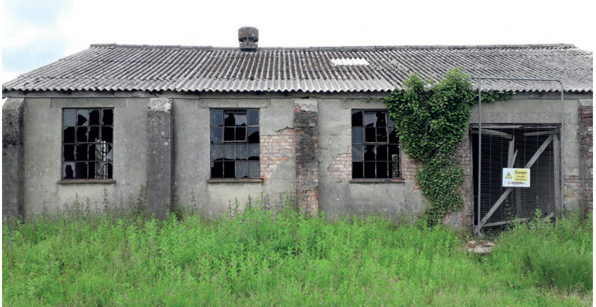
The Generator Building at Stow Maries
