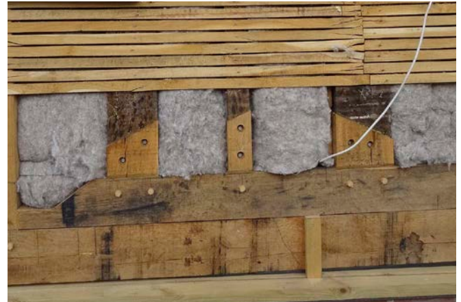
Insulation in timber-framed wall
