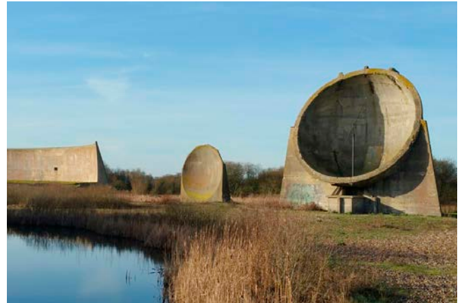
Concrete sound mirrors in Dungeness, Kent
