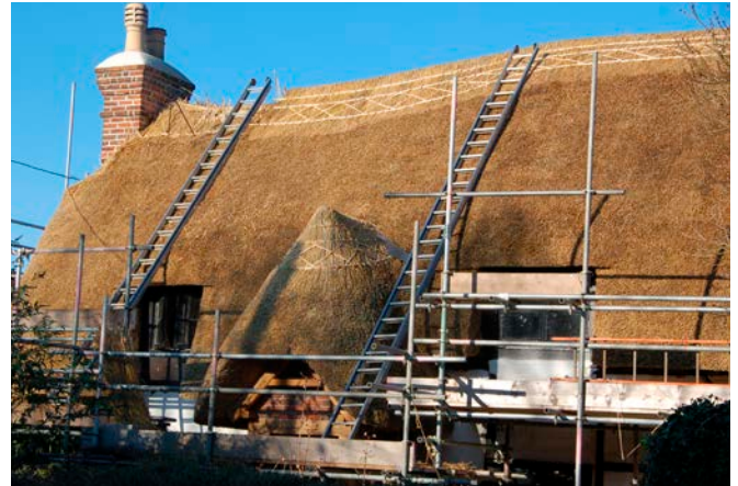
Re-thatching a cottage
