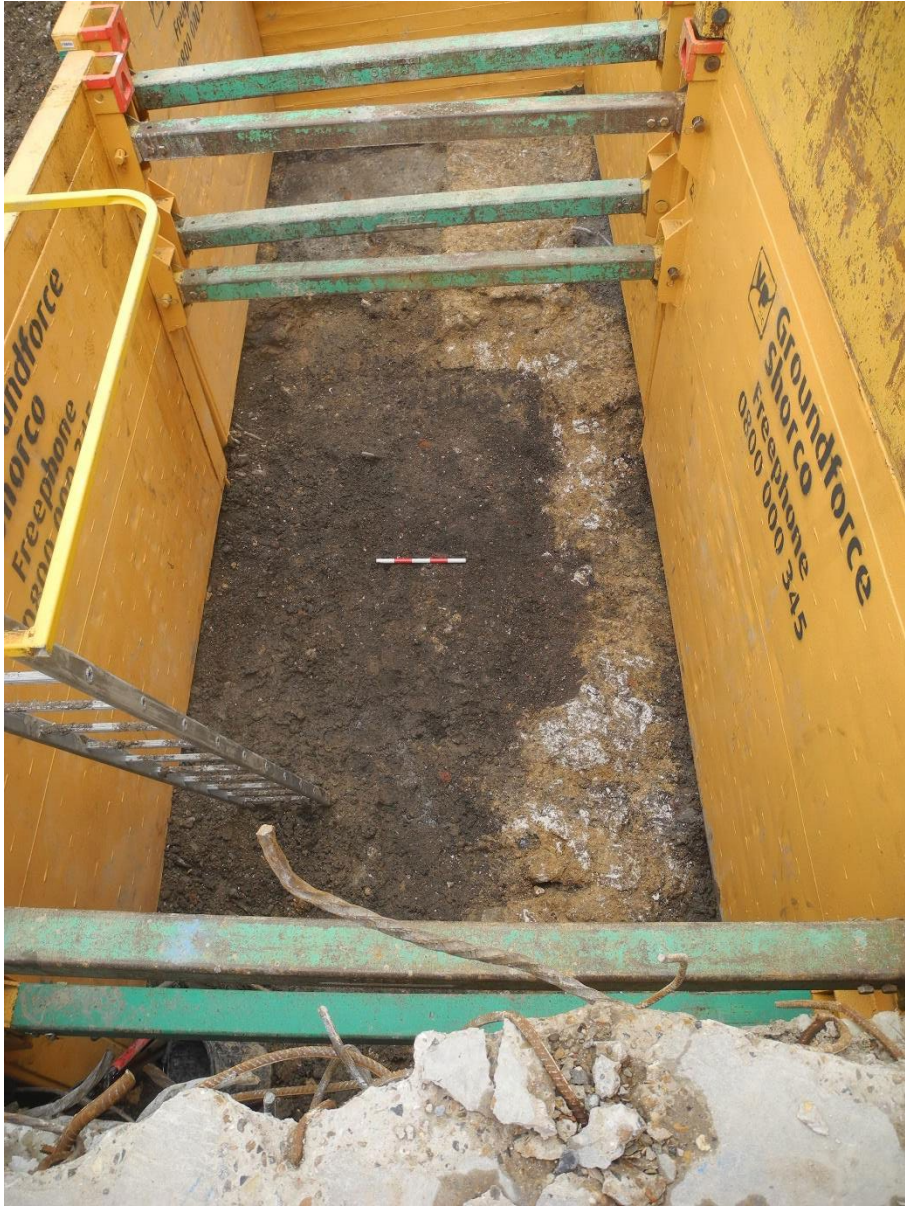
Medieval chalk foundation in base of trench Copyright MOLA 2024
