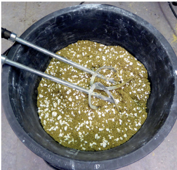
Small batches of hot mixed mortar can be mixed by hand or using a hand-held paddle mixer. Larger volumes can be made in a forced-action mixer or roller-pan mixer.
