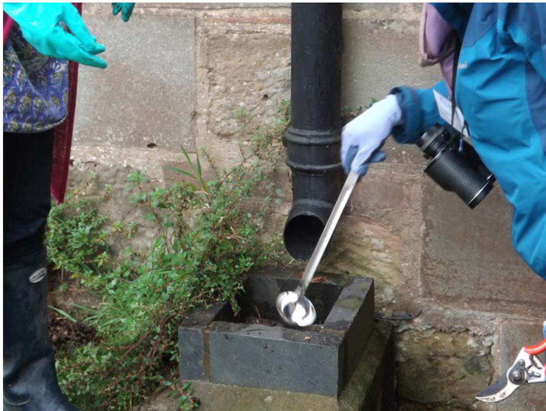
Co-op volunteers clearing a blocked drainage gully (Photo: SPAB).
