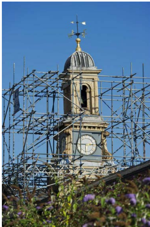
Clock Tower at Green Lane Works © Historic England
