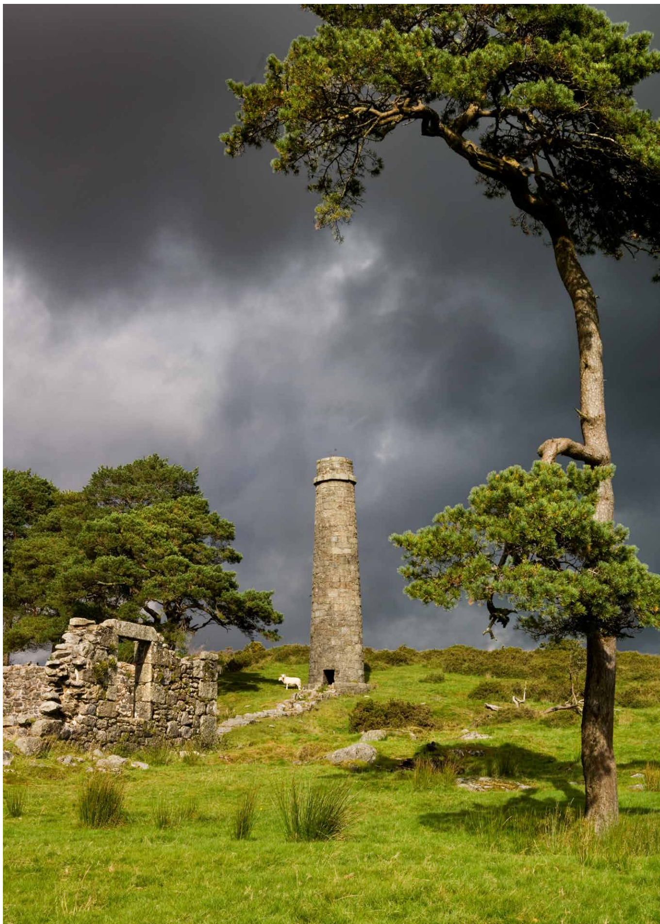
Remains of the Powder Mills at Postbridge, Dartmoor, Devon. Showing chimney and ruined building against an overcast sky. © Historic England Archive
