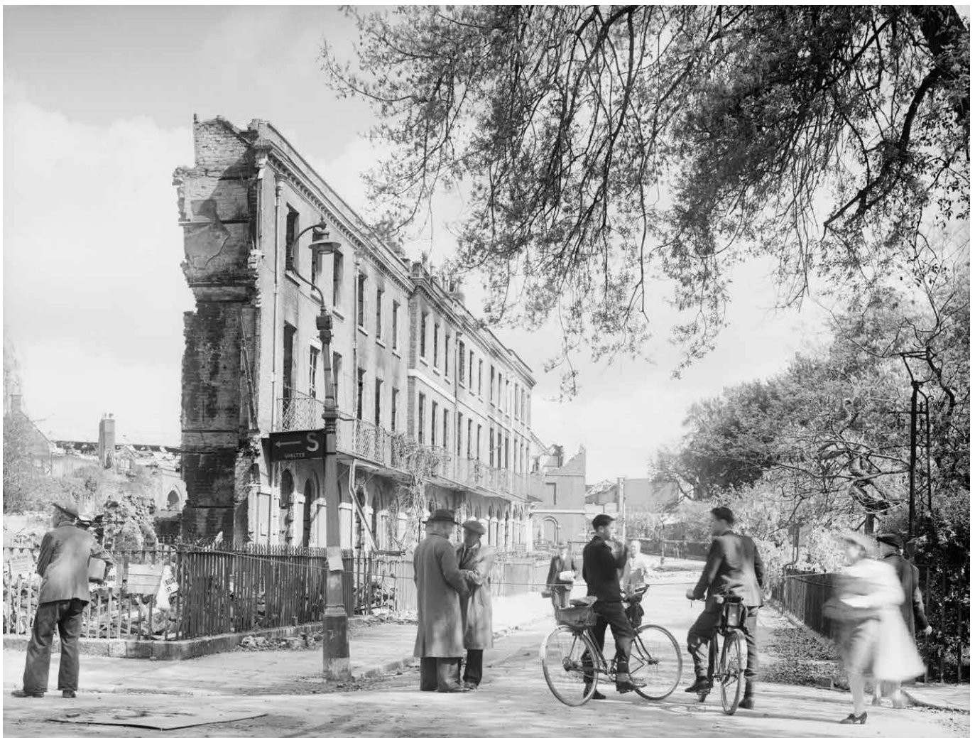
The facade of 25-36 Southernhay West, Exeter, Devon. Photographed by Margaret Tomlinson after an air raid in 1942. © Historic England Archive
