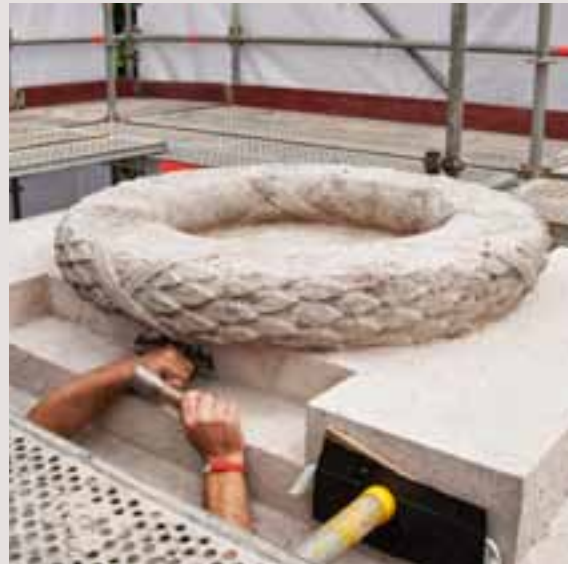
Conservation works in progress (left and bottom left)
