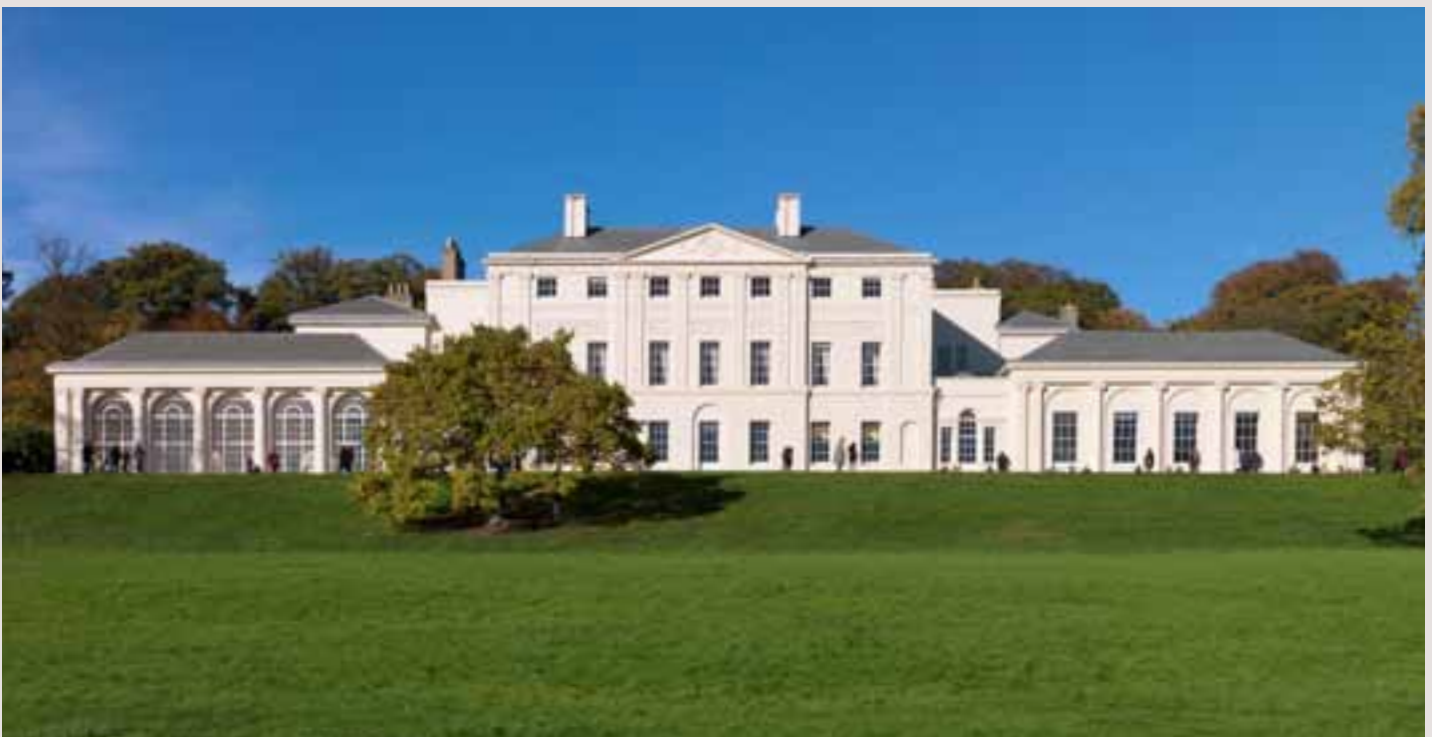
The south front of the house
