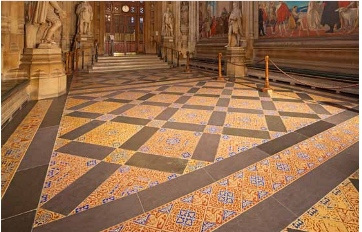
The newly reinstated floor to St Stephen's Hall
