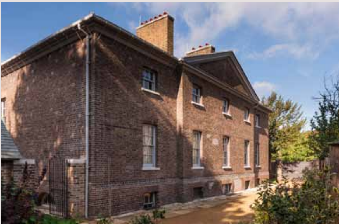
East elevation of the royal kitchens
