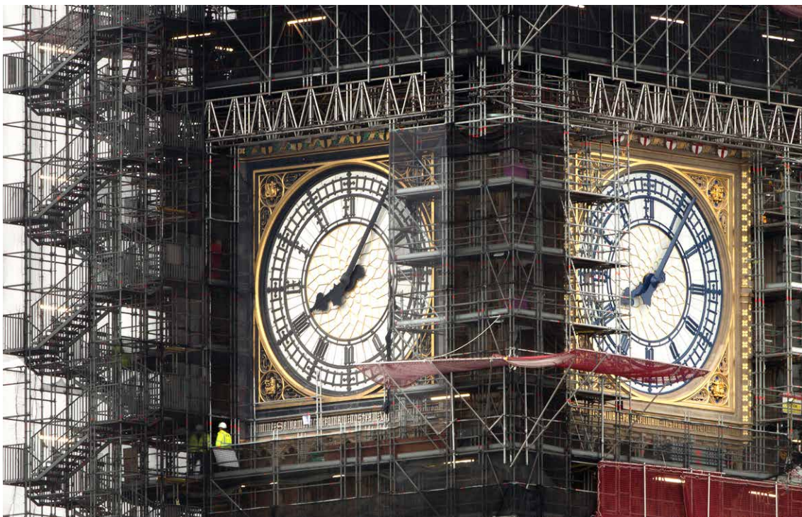
The Elizabeth Tower of the Palace of Westminster showing the east dial (left) before conservation, and the north dial (right) following cleaning, repairs and reinstatement works. © UK Parliament / Adam Watrobski
