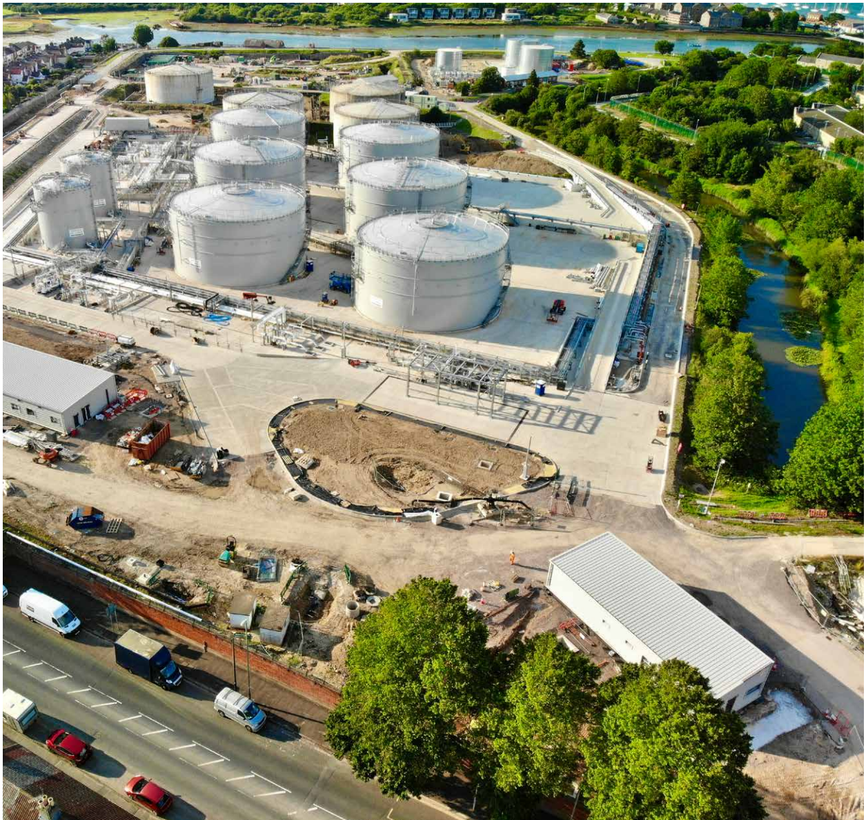
Gosport Oil Fuel Depot, established in 1907, has had its fuel tanks replaced with archaeological advice and survey provided by the Defence Infrastructure Organisation. © The Oil and Pipelines Agency
