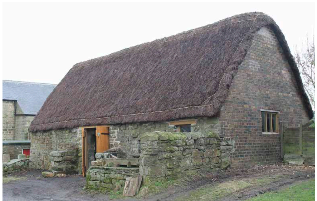
Figure 4: Black Barn after the conservation works
