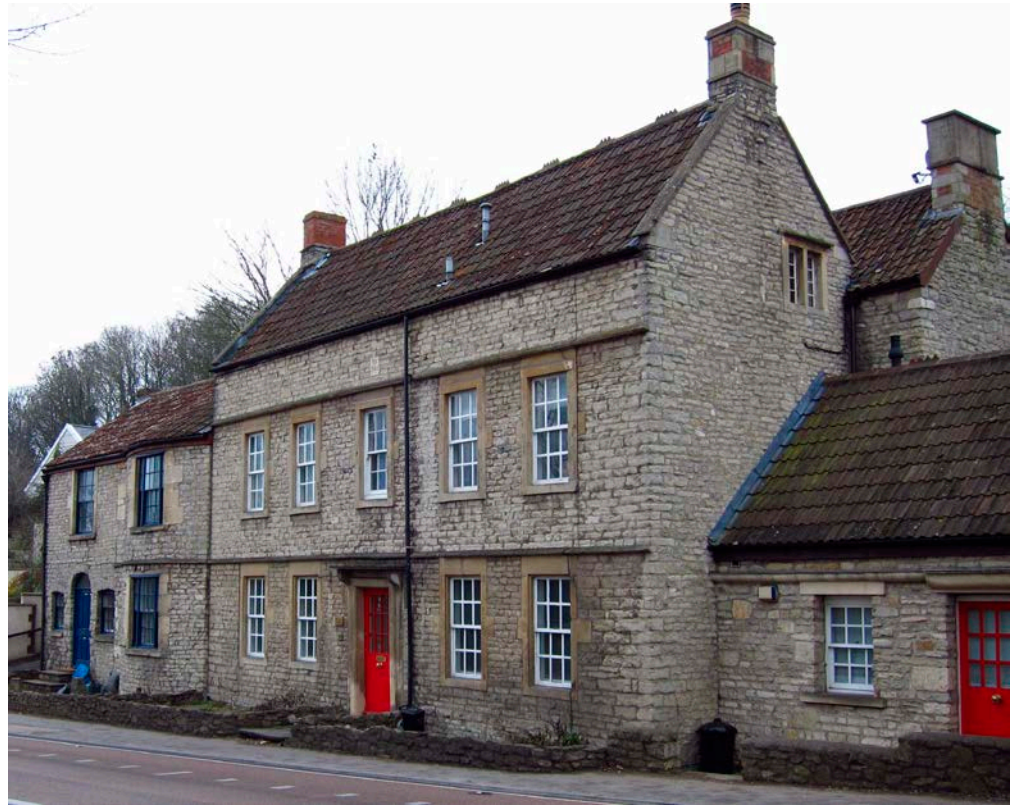
Figure 22: Houses, Bath Road, Saltford. Saltford Stone.
