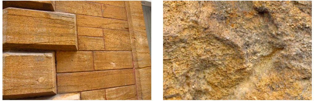
Figure 28: Twinhoe Beds stone details.
