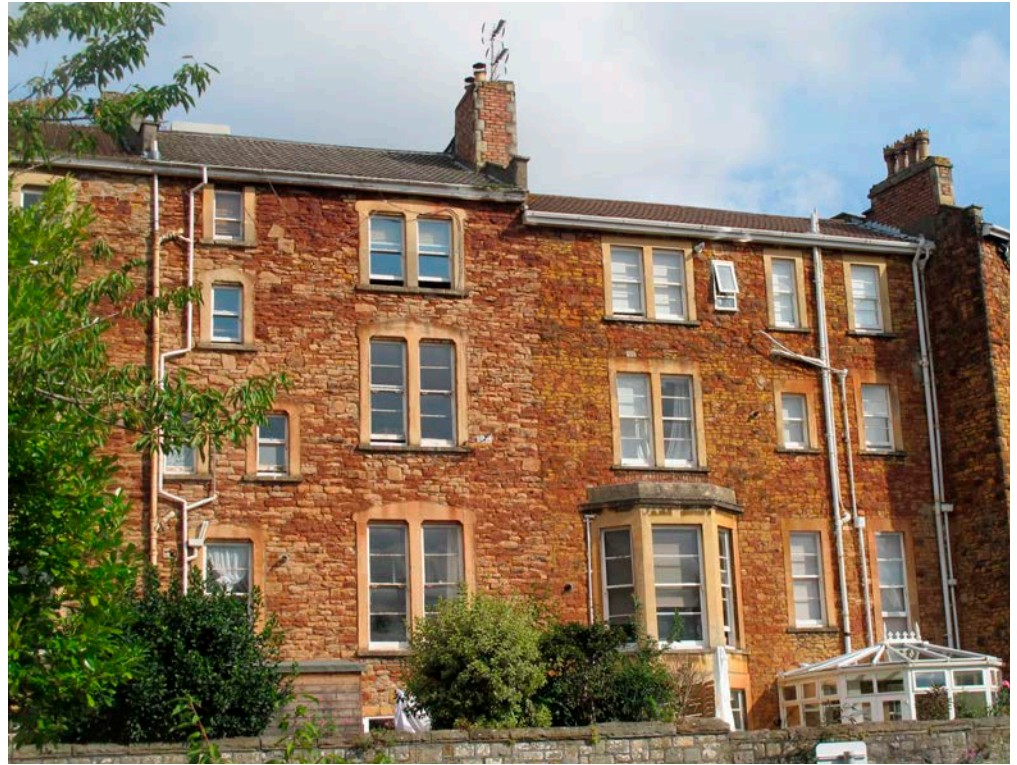
Figure 13: Terrace houses and walls, Whatley Road, Clifton, Bristol. Dolomitic Conglomerate.
