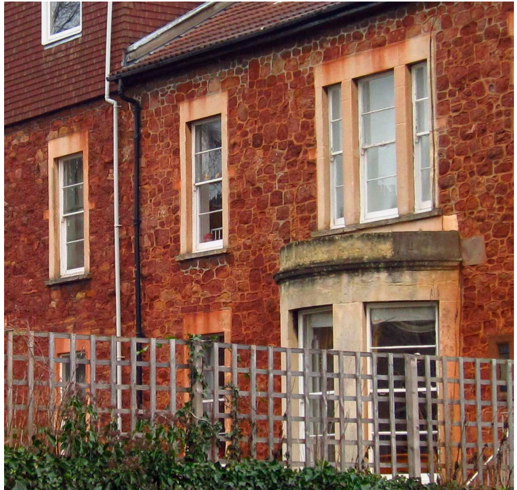
Figure 16: Houses, Fairview Drive, Redland, Bristol. Redcliffe Sandstone and Dolomitic Conglomerate.
