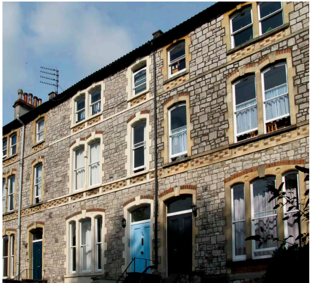
Figure 7: Terrace houses, Chandos Road, Redland, Bristol. Lower Carboniferous Limestone.
