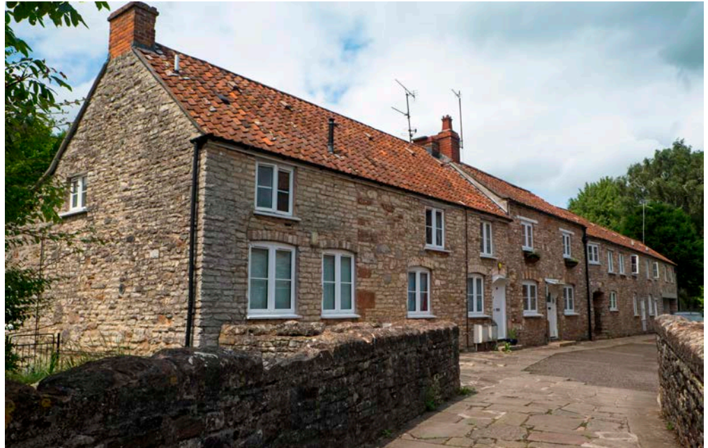
Figure 17: Cottages, The Street, Chew Stoke. Skerry Sandstone and Butcombe Sandstone.
