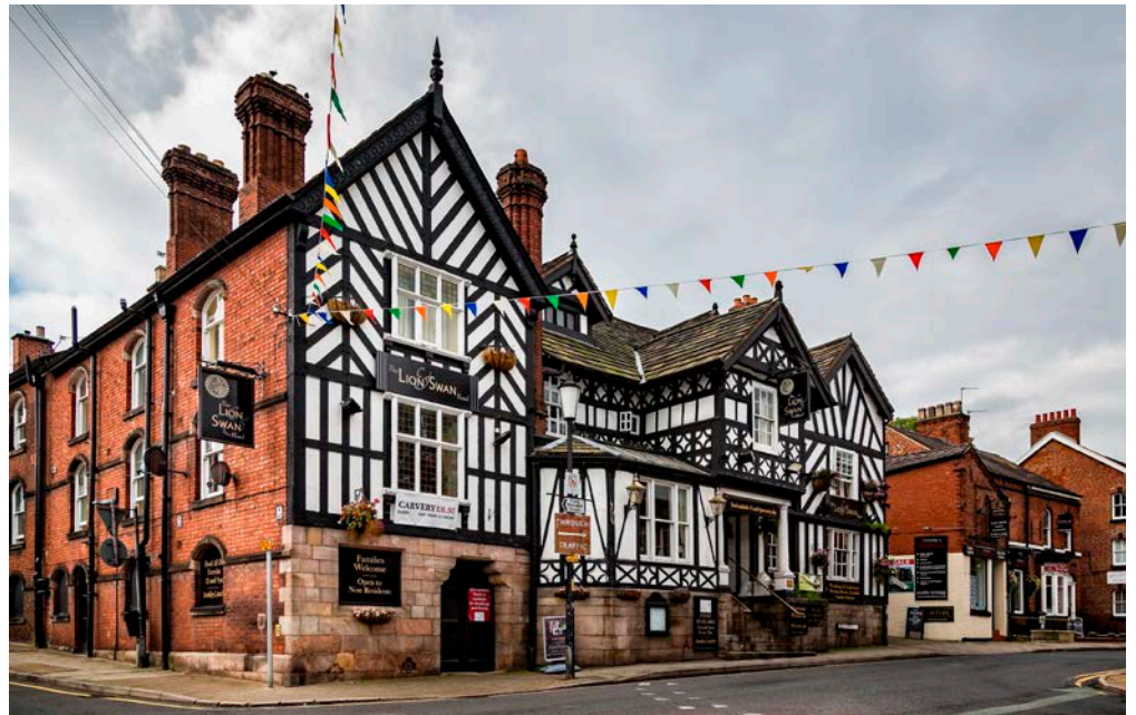
Figure 4: The Lion and Swan, Congleton. Rough Rock used for plinth and lower levels.
