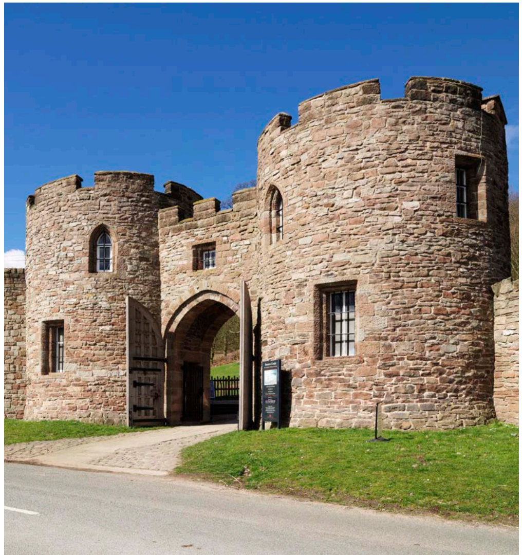
Figure 9: Beeston Castle, Beeston. Sandstones from the Passage Beds and Delamere Sandstone Member.
