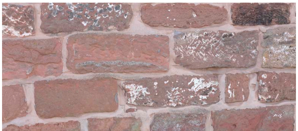
Figure 15: Outbuildings on Bellemonte Road, Frodsham. Frodsham Sandstone.
