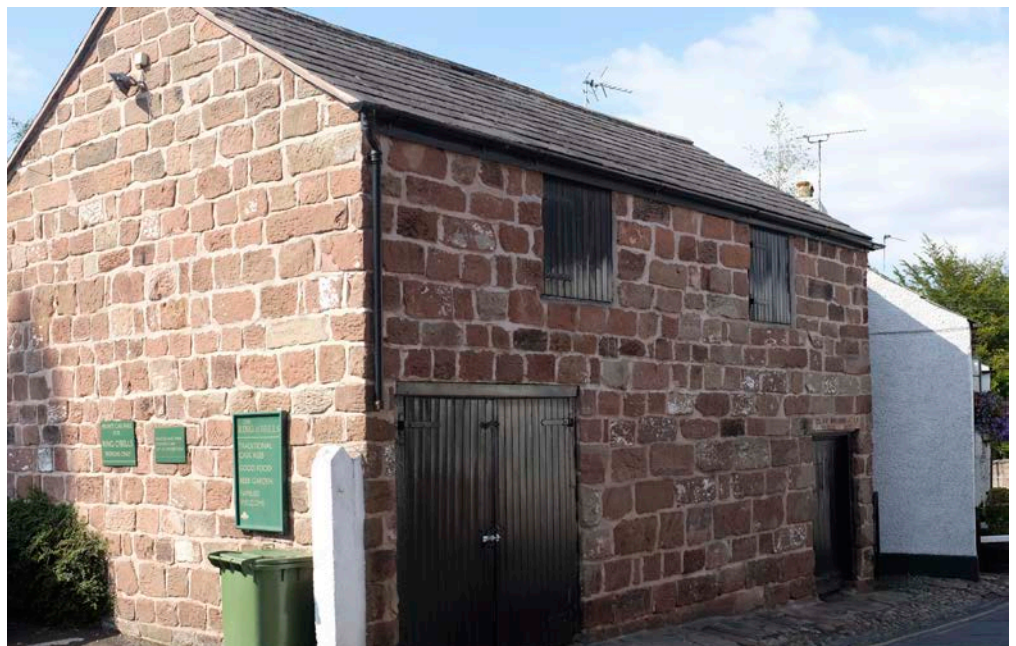
Figure 14: Outbuildings on Bellemonte Road, Frodsham. Frodsham Sandstone.
