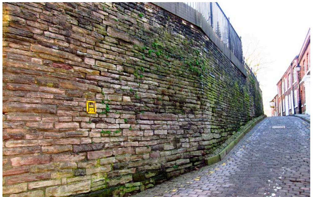
Figure 5: The wall adjoining the Church of St Michael and All Angels, Macclesfield. Rough Rock.
