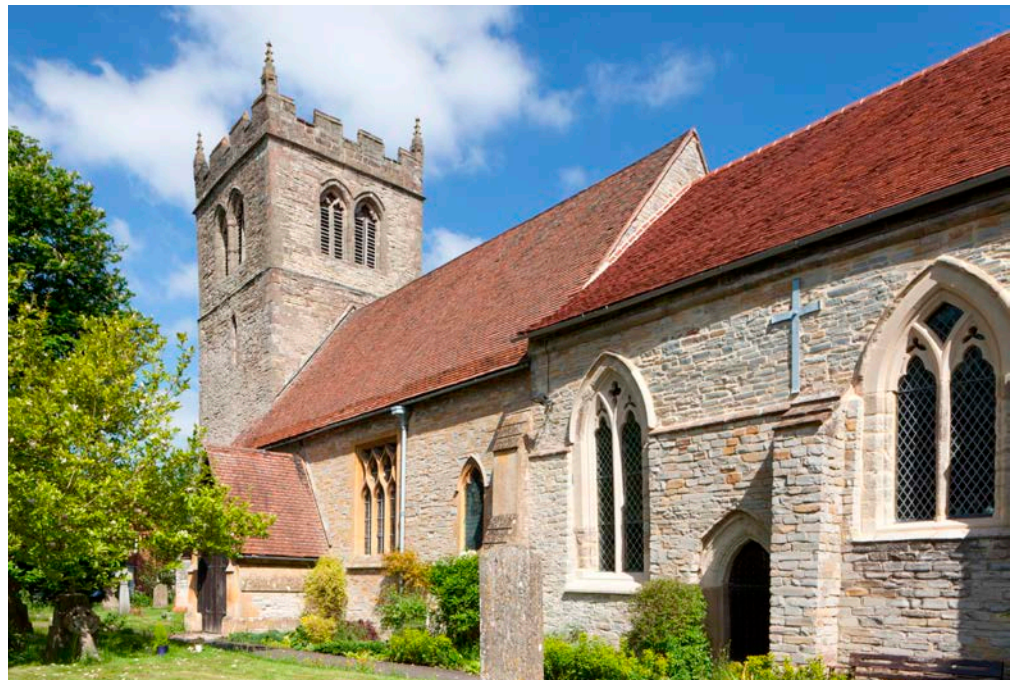
Figure 15: Church of St John the Baptist, Aston Cantlow. Wilmcote Sandstone with window mouldings in Arden Sandstone.
