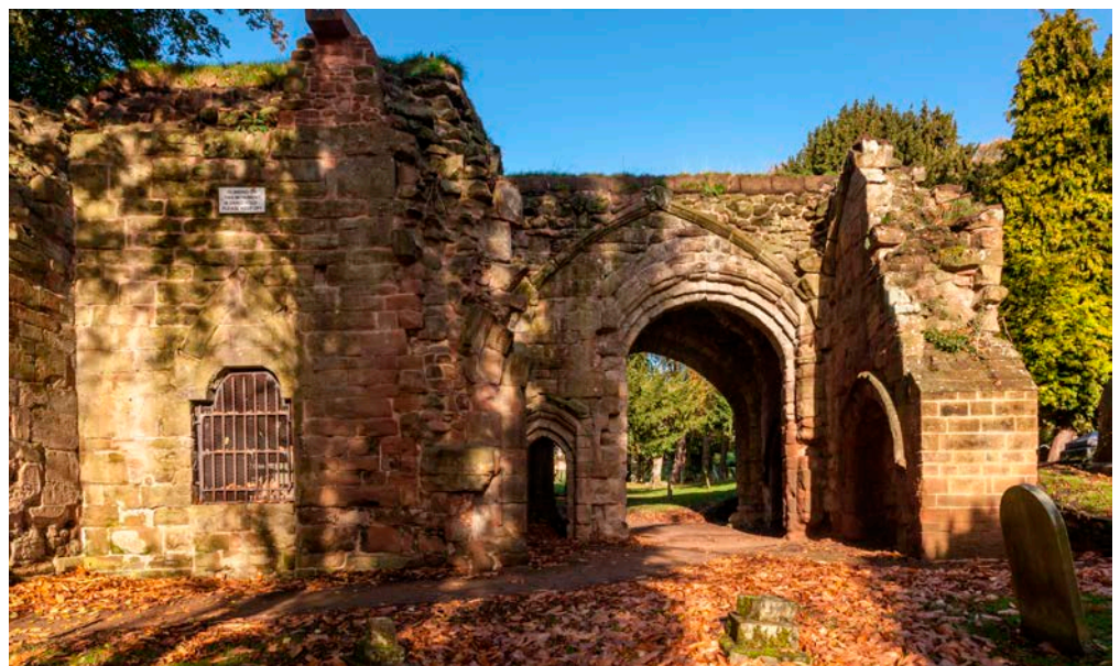
Figure 6: Abbey gatehouse, Kenilworth. Kenilworth Sandstone.
