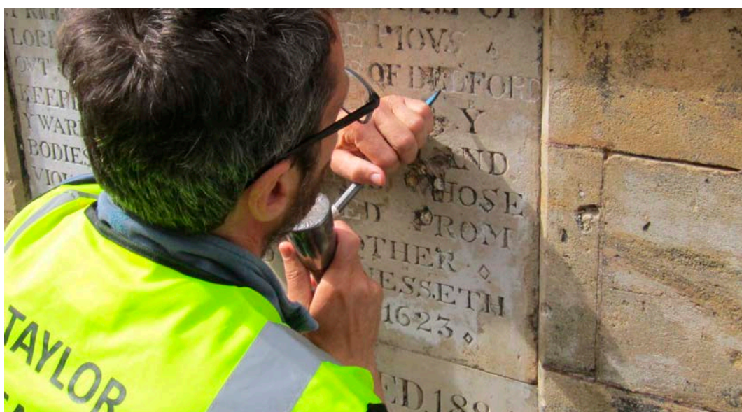
Figure 24: An experienced letter cutter can sharpen the inscription on a deteriorated stone panel to improve its legibility.
