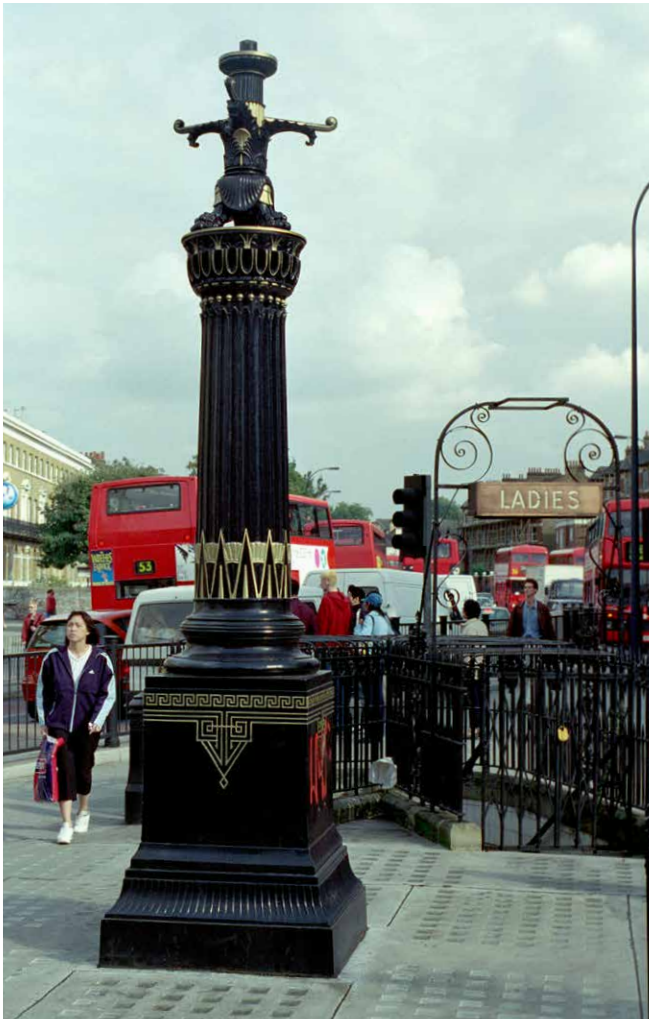
Figure 3 A rare combined ventilating pipe and gas lamp in New Cross Road, London (listed Grade II), installed 1897 as part of public conveniences for Greenwich District Board of Works. The ventilating pipe extracted foul gases from the lavatories below, to be burnt off by the gas mantle at the top. The Egyptian-pattern ventilating column was made by Macfarlane's Castings of Glasgow, to a design by Alexander 'Greek' Thomson.
