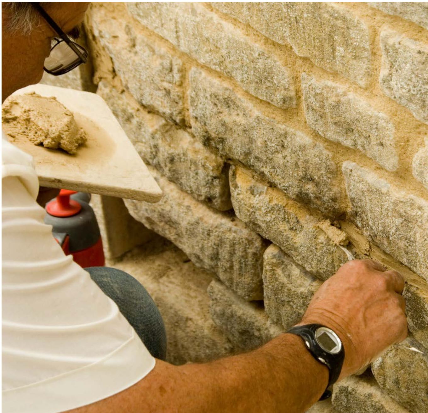
Above: Lime mortar is applied between stones.
