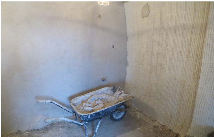
Left: Insulated lime plaster applied directly to a masonry wall.
