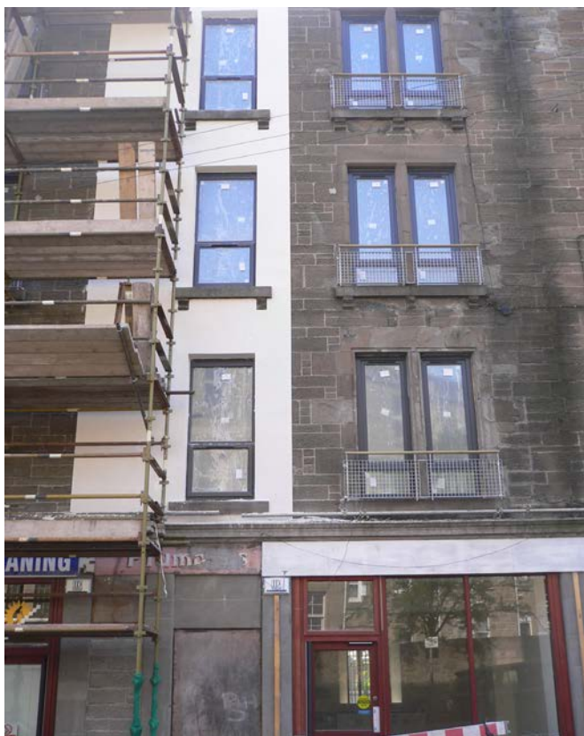
Left: Contrast between part of a building with external wall insulation and part that has none. The visual impact is considerable.
