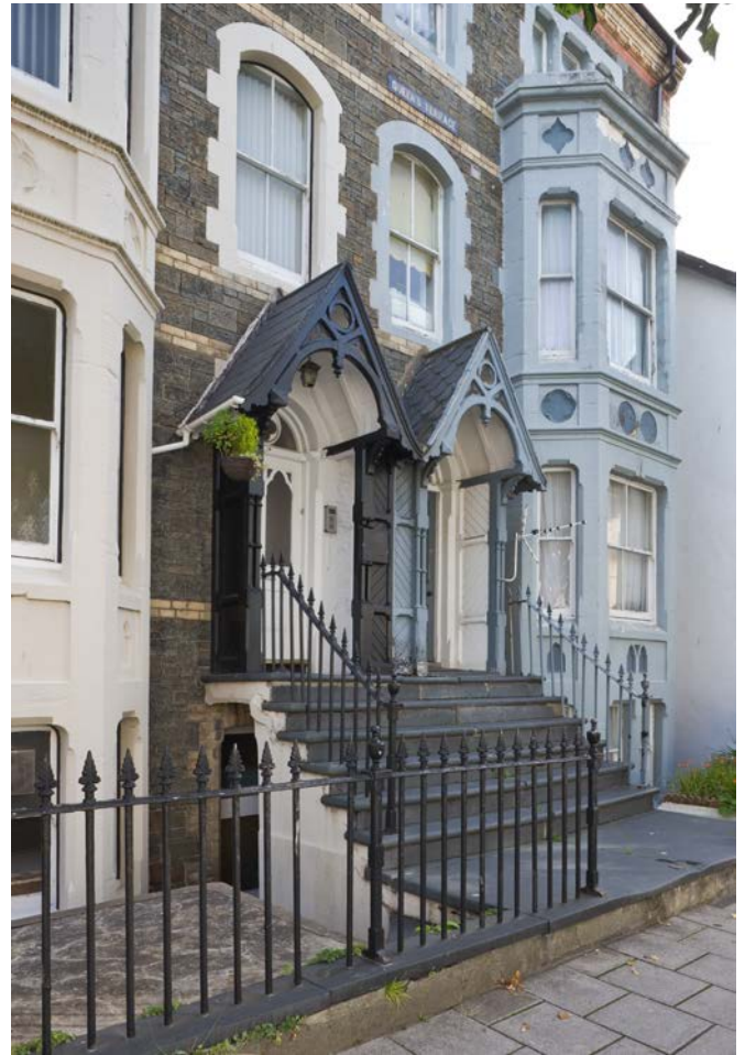
© Crown copyright: Royal Commission on the Ancient and Historical Monuments of Wales
