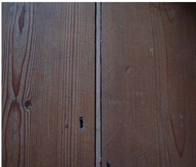
Left: Plugging gaps between floorboards.
