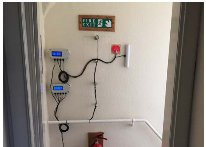
Above: Continuous hygrothermal monitoring setup.
