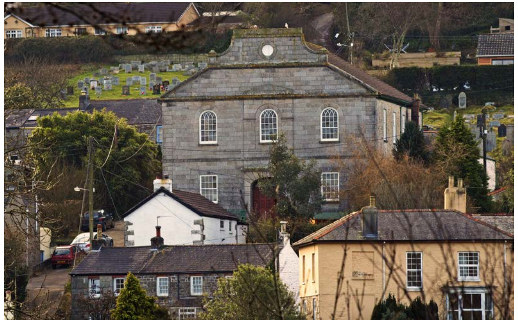
Figure 3: The large classical Wesleyan chapel of 1843 at Ponsanooth (Grade II*) dominates this former industrial village. © Eric Berry
