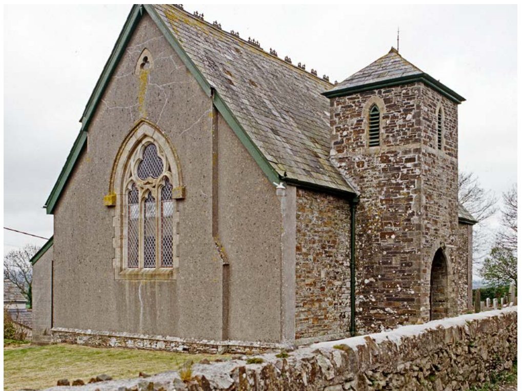
Figure 21: The 1873 chapel of St Thomas the Apostle at Tregadillet is one of a small number of Methodist chapels in Cornwall with a bell tower. © Eric Berry
