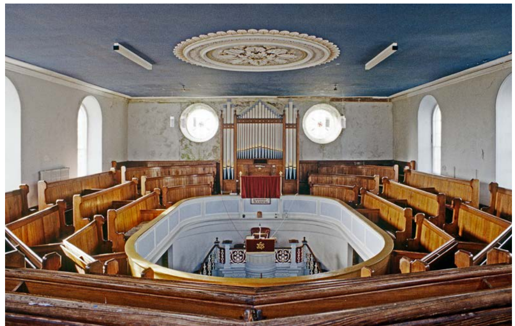
Figure 29: The interior of the 1862 Wesleyan chapel at Leedstown in Crowan parish (Grade II) has an original gallery. However, as with so many Methodist chapels, the building was re-seated in the late-19th century with simple pitch pine pews. Attention is still focused on the fine original ceiling rose and also drawn to the late 19th century rostrum that may incorporate the bow front of the original pulpit.
