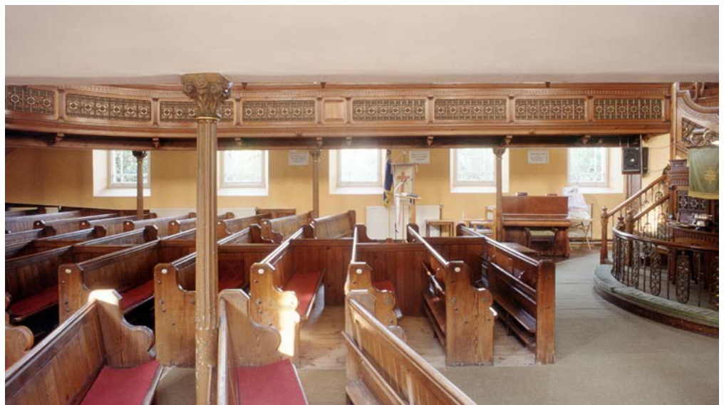
Figure 37: The interior of the 1858 unlisted chapel at Bugle was completely remodelled and refitted in 1890. The pitch-pine pews are of a standard design, with v-jointed boards and shaped ends with ceramic numbers, but the richly decorated panelled and pilastered gallery front is emphasised by its architectural treatment. © Eric Berry
