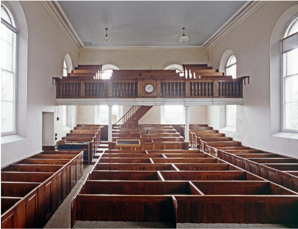
Figure 28: View towards the end gallery (inserted c.1881) of the former c.1868 Wesleyan chapel at Little Trethewey (Grade II*), St Levan, showing the cast-iron columns on which it is supported and the balustraded front. The rare box pews are ramped up at the rear to enable a view of the rostrum. The rostrum end of the chapel was refitted when the chapel was extended in 1895 at Tuckingmill.
