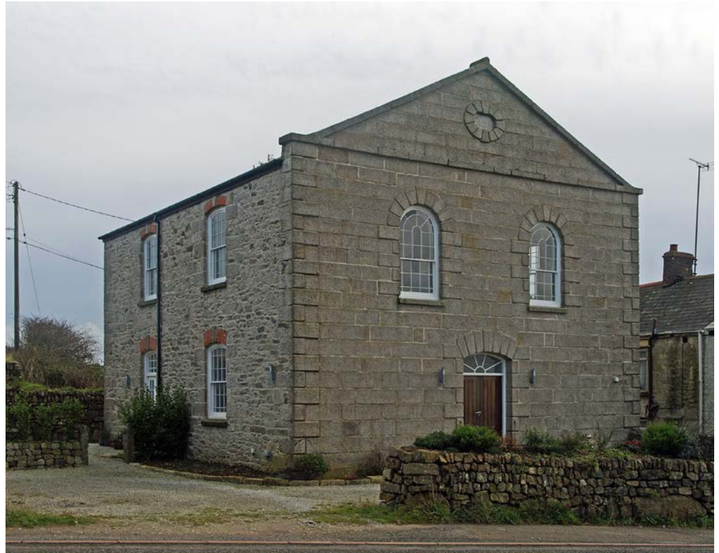
Figure 16: The former Wesleyan chapel at Manhay (Grade II) in Wendron parish has a fine pedimented ashlar façade, with rusticated surrounds to the door and sash windows lighting the gallery. The building has now been converted to a house but retains its external character. © Eric Berry
