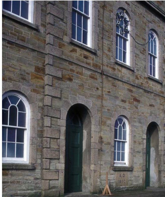
Figure 22: Panelled doors with fanlights and hornless sash windows, as exemplified within the 1860 pedimented façade of the Wesleyan chapel at St Agnes (Grade II). © Eric Berry
