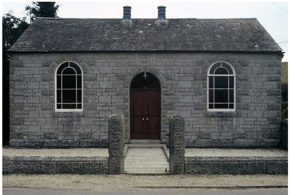
Figure 11: The side-entry chapel at Lowertown, Wendron (1887) replaces an earlier former chapel (now a ruin). Classical detail – in this case rusticated stonework to the quoins and openings – has been applied to a simple symmetrical elevation. © Eric Berry
