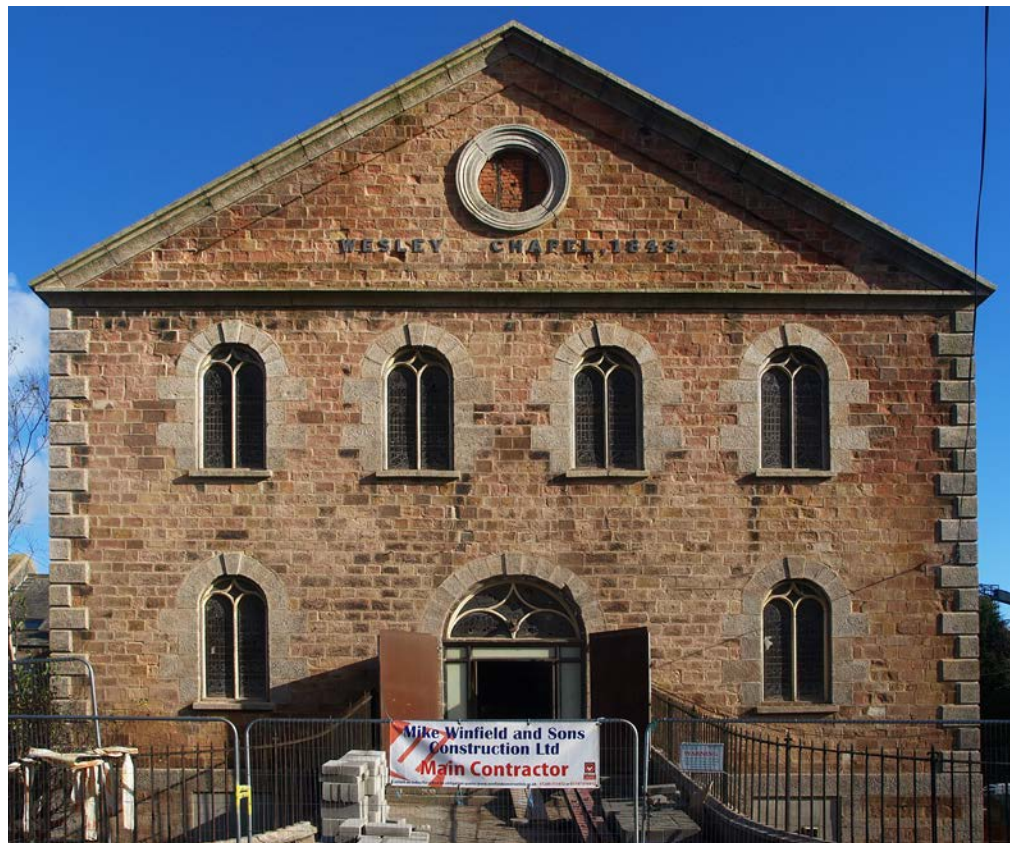
Figure 25: By the end of the 19th century windows were being installed with paired lights and a roundel, either in a pointed-arched or round-headed opening. These windows were inserted within the original openings of the 1843 (Grade II) Classical chapel at Tuckingmill. © Eric Berry
