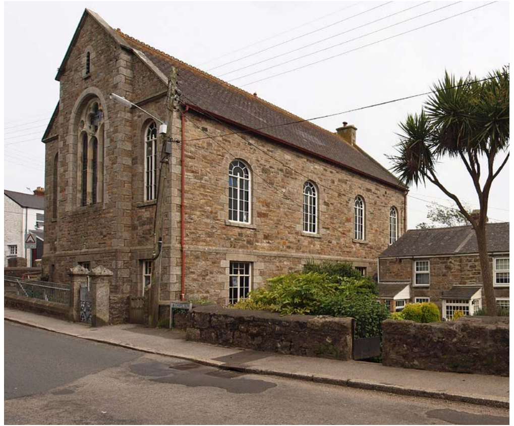
Figure 42: The 1884 former Wesleyan chapel at Gulval (Grade II), now a studio, exemplifies a design type where the Sunday School and other rooms are accommodated within a basement underneath the chapel. © Eric Berry
