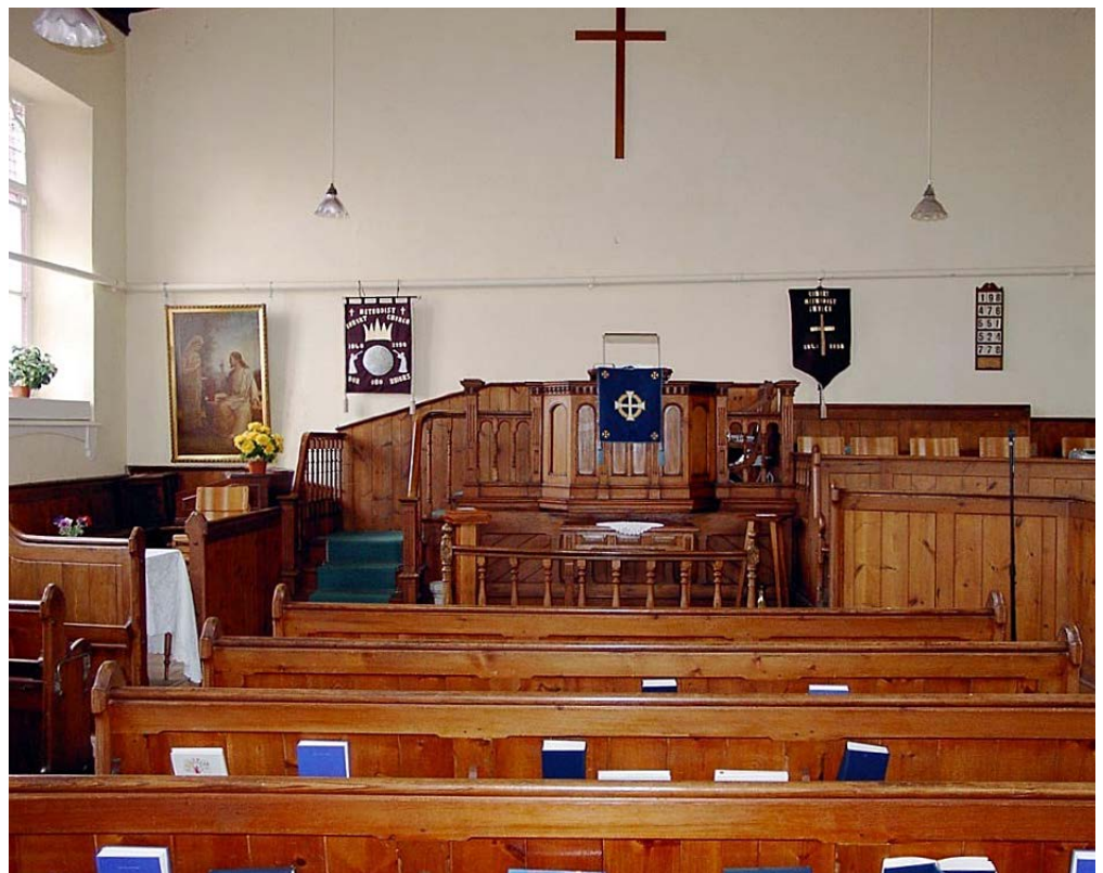
Figure 27: The former 1849 Wesleyan chapel at Cubert (Grade II), now closed, was refitted in the late-19th century. The pews and rostrum were of varnished pitch-pine, which is characteristic of this period. The layout of the pews either side of the rostrum possibly repeats the original pew arrangement and includes a choir or musicians’ area, or possible former leaders’ pews. © Eric Berry
