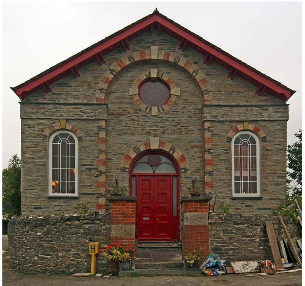
Figure 15: The gabled façade to this chapel (opened 1874) at Tredrizzick has a recessed central bay rising to an open pediment. Its show front, with the central bay and entrance picked out in coloured brickwork, is almost identical to that of the 1869 chapel at St Tudy (Grade II). © Eric Berry
