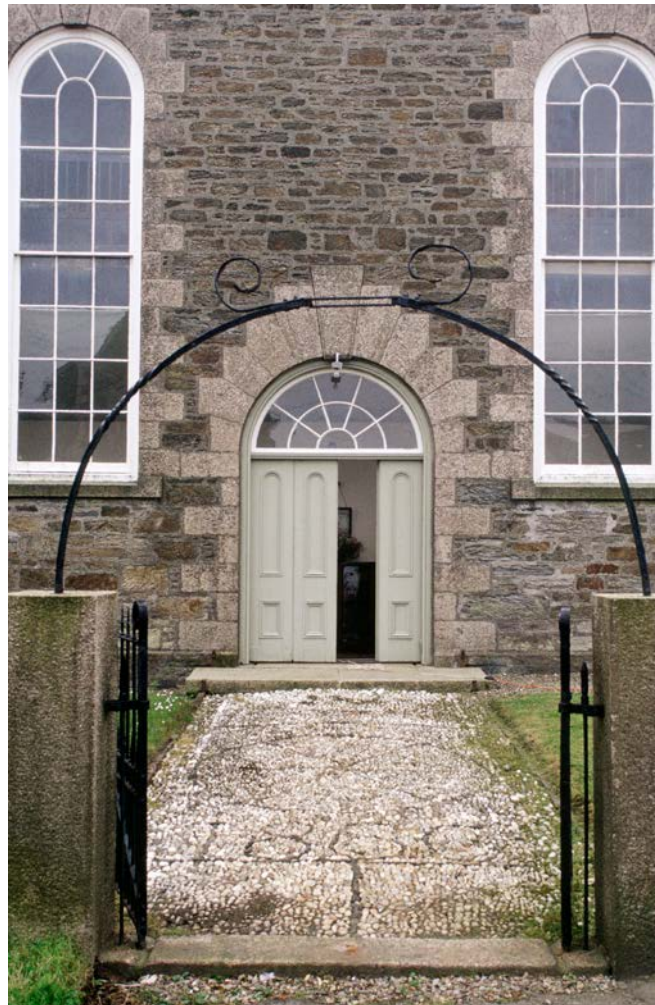
Figure 48: The former Wesleyan chapel at Voguebeloth in Illogan (Grade II*) has a foundation stone of 1865 and the date 1866 picked out in the cobble pathway. © Eric Berry
