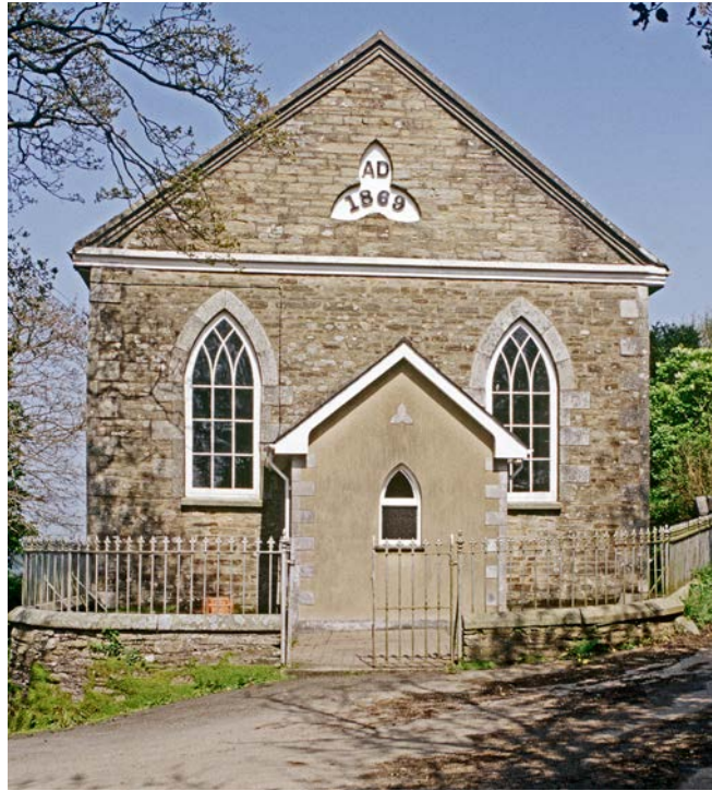
Figure 24: The windows of the 1869 chapel at Porthkea (Grade II) are distinctive examples in the 18th century Picturesque Gothic style, with intersecting glazing bars. © Eric Berry
