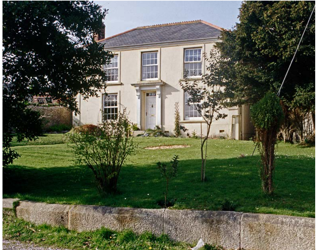
Figure 46: At Carharrack the former manse (Grade II) is sited close to the 1815 chapel (Grade II*). © Eric Berry
