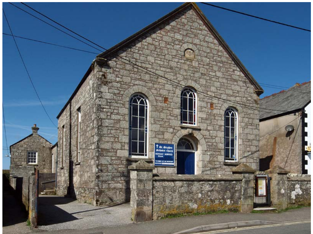
Figure 17: The Wesleyan chapel at St Stephen in Brannel (1870, Grade II), is one of a group of similarly-designed chapels, built into the 1870s, in this china clay district west of St Austell. © Eric Berry
