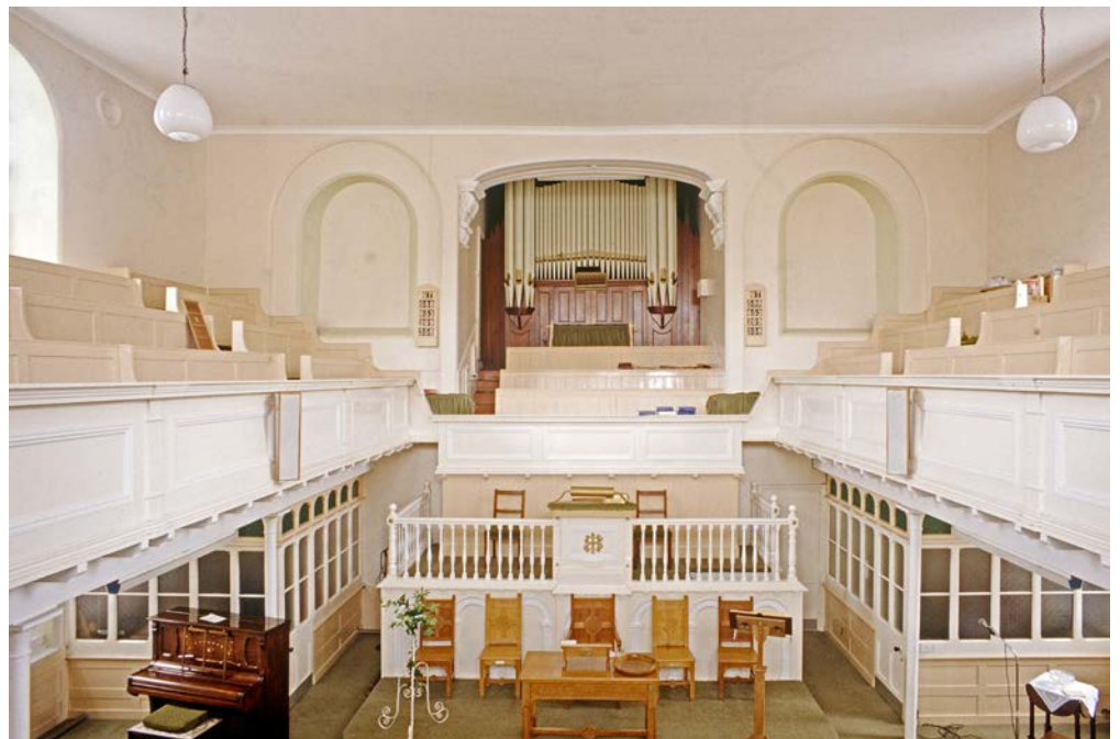
Figure 31: The galleried United Reform (originally Bible Christian) chapel at Berkeley Vale, Falmouth (Grade II*) has a fine interior with original box pews and large balustraded rostrum. Leaders' pew areas to either side of the rostrum have been screened off at a later date. © Eric Berry
