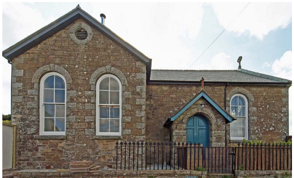
Figure 23: Horned sash windows are marked by projecting lugs, which help to strengthen the meeting rails in combination with the heavier glass used from the mid-19th century. They are a type commonly used from the 1870s in Cornwall. This is the (unlisted) late chapel at Newbridge in Sancreed parish. © Eric Berry
