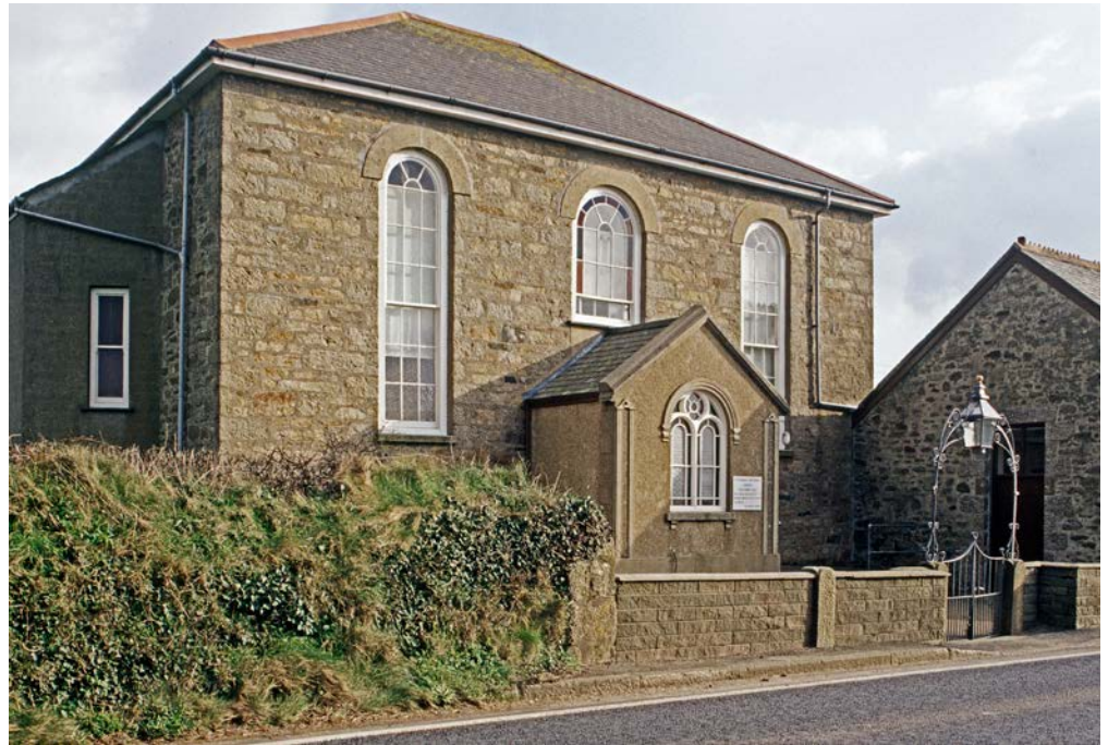
Figure 10: The rather unusual mid-19th century chapel at Trewennack in Wendron parish has round-arched sash windows set into stone rubble walls. The roadside elevation was fitted with a later central entrance porch so that the later Sunday School (right) was accessed from the roadside forecourt. © Eric Berry
