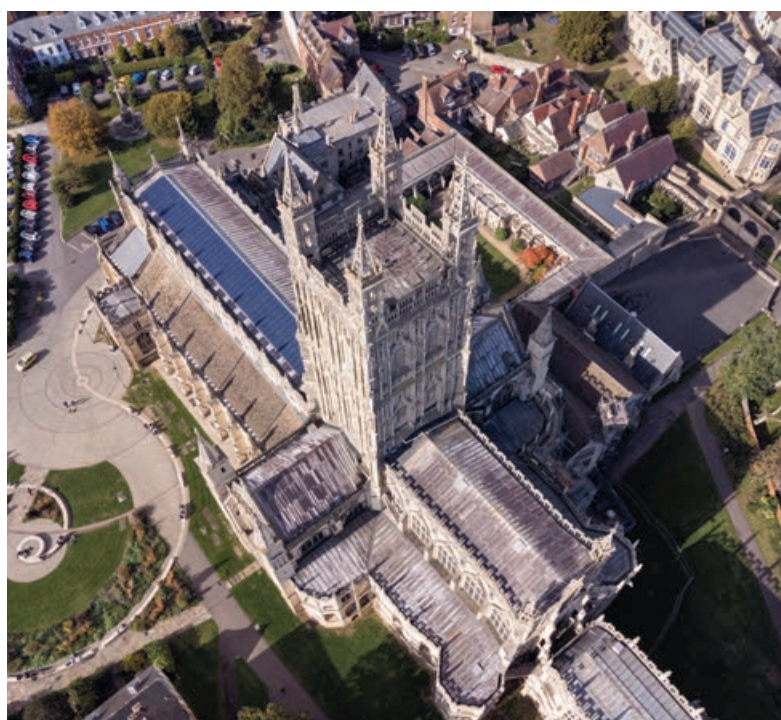
Solar panels on the nave roof of Gloucester Cathedral, College Green, Gloucester
