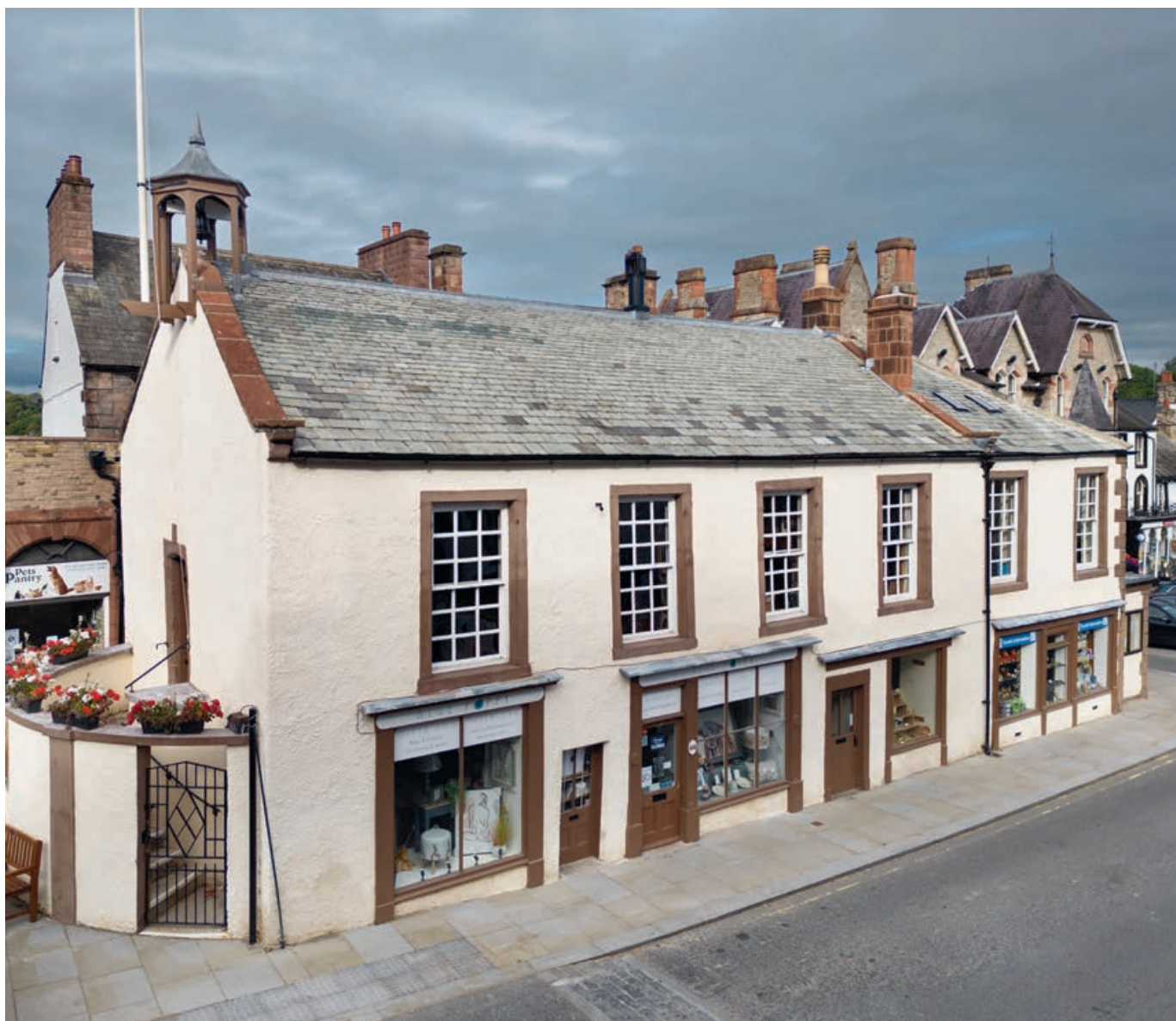
The newly renovated Moot Hall, Appleby. Work was carried out as part of Appleby Heritage Action Zone
