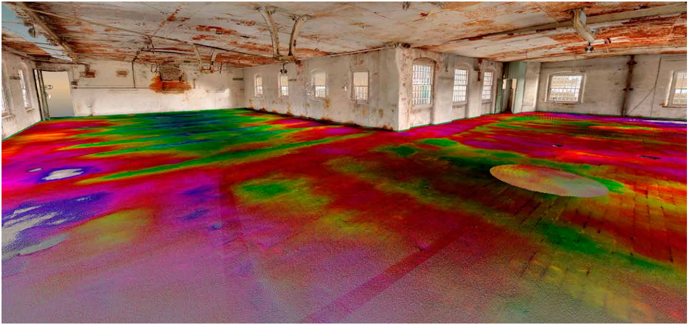
Long Mill, Darley Abbey: laser survey showing in red/magenta the slight pathways on the floor eroded between machine locations, which are shown in green/blue. © Derbyshire County Council
