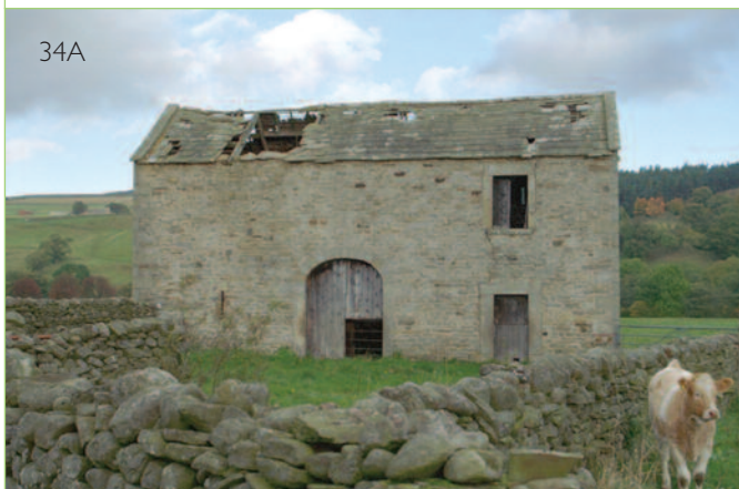
34 Outfarms and field barns in the North East Region Outfarms, with buildings providing a threshing barn and stock housing, often with a fold yard (A) and field barns consisting of a cow house
