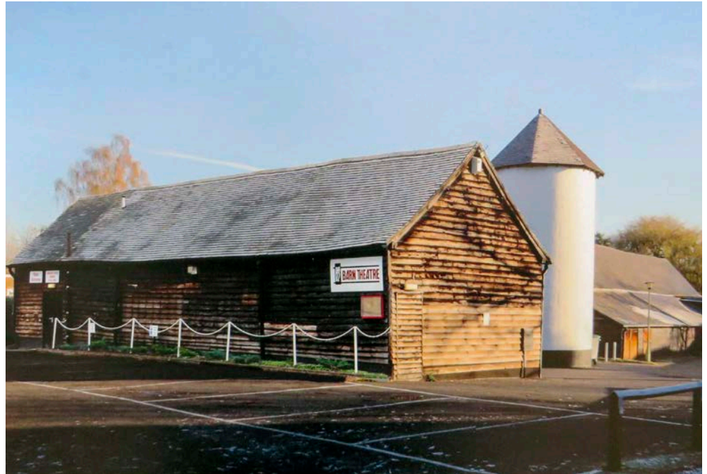
Figure 17: Concrete silo and feather-edged weatherboarding to the 17th century timber-framed Welwyn Barn Theatre, a converted cowshed. Listed Grade II.
