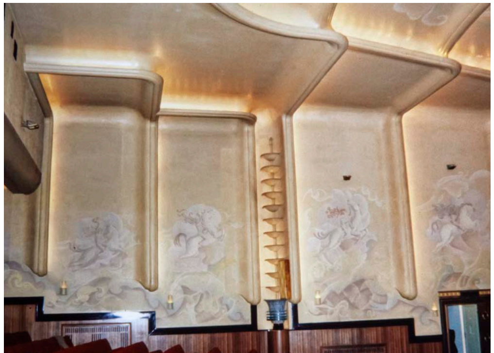
Figure 18: Auditorium side wall and ceiling of Stanford Hall Theatre are divided into staggered sections by a series of lighting covers, with murals on each leaf and full height central Art Deco uplighter. Listed Grade II*.
