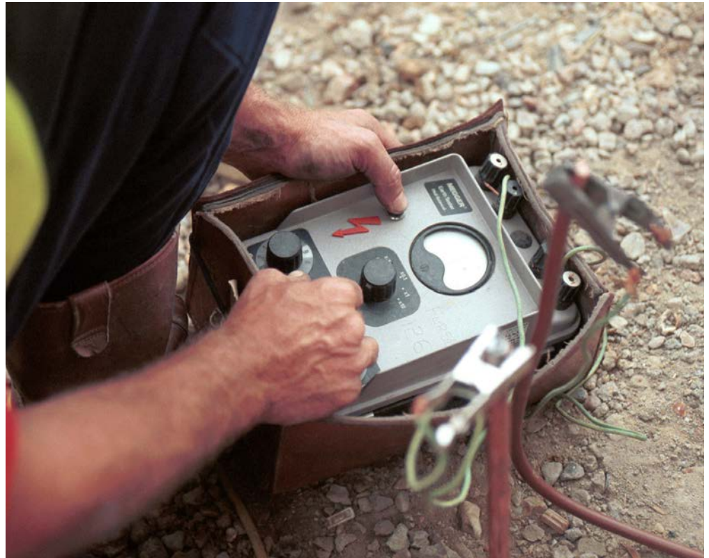
Figure 24: Engineer testing an installation.
