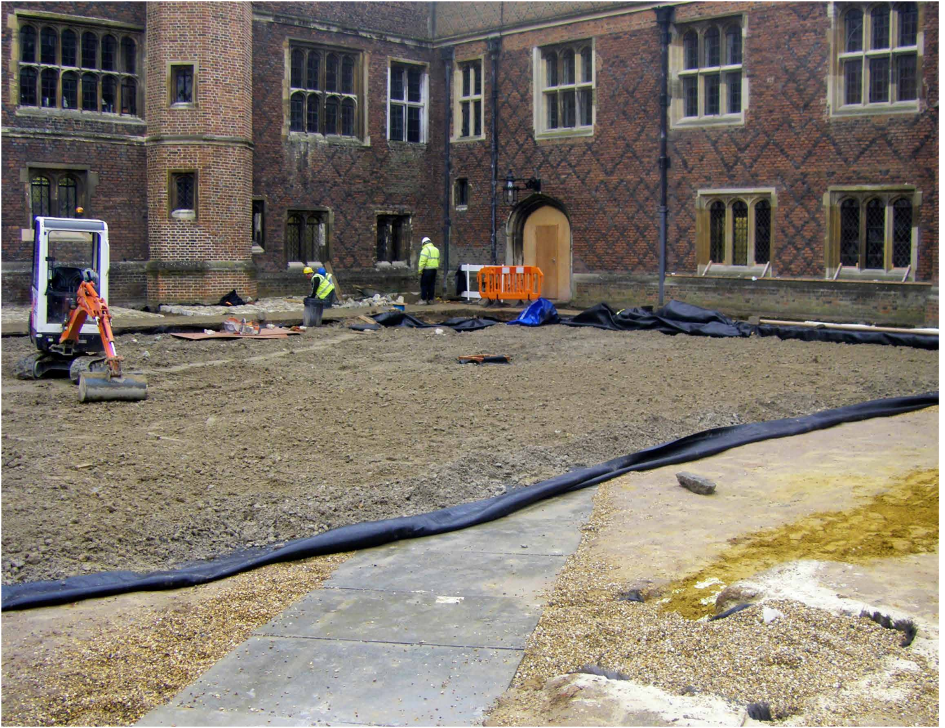
Figure 7 General geotextile cover and final base layer.
