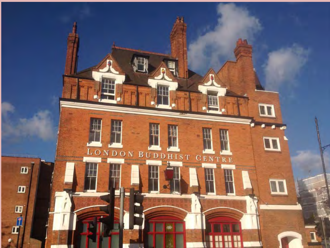
Former Bethnal Green Fire Station source: authors' own
