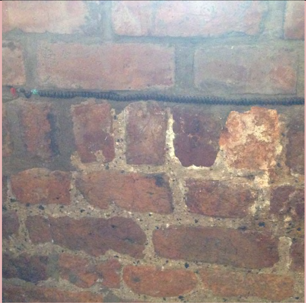
A mala (string of beads) cemented between the bricks
