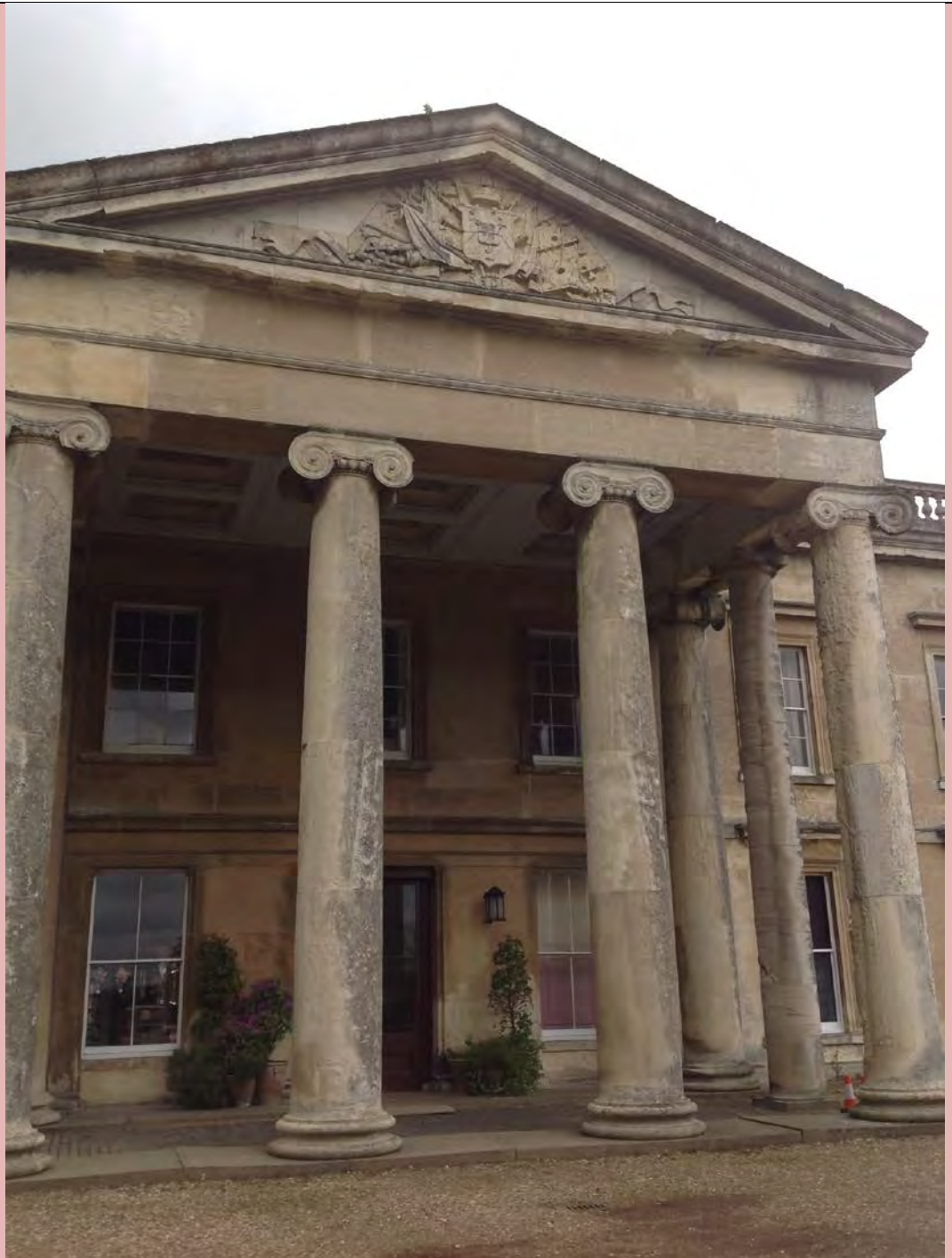
The entrance to Kilwick Percy Hall
