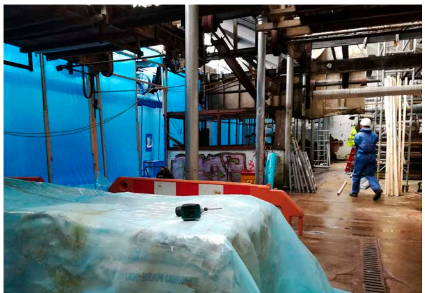
Figure 19: Asbestos decontamination works in progress, 2021. © Vanessa Ruhlig
