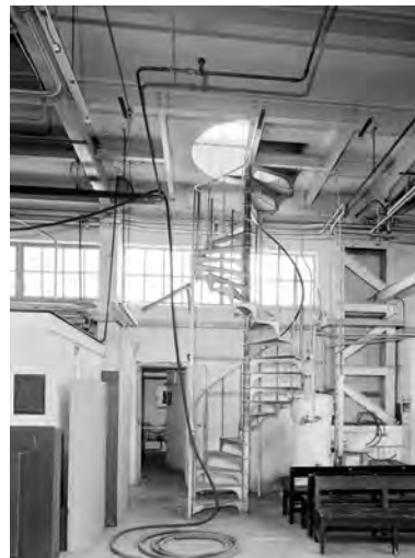
Fig. 245. BB97/09263. Photograph of the spiral staircase in north end of Boathouse No. 4, Portsmouth (28 Jul 1997). ©Crown copyright.HE.
