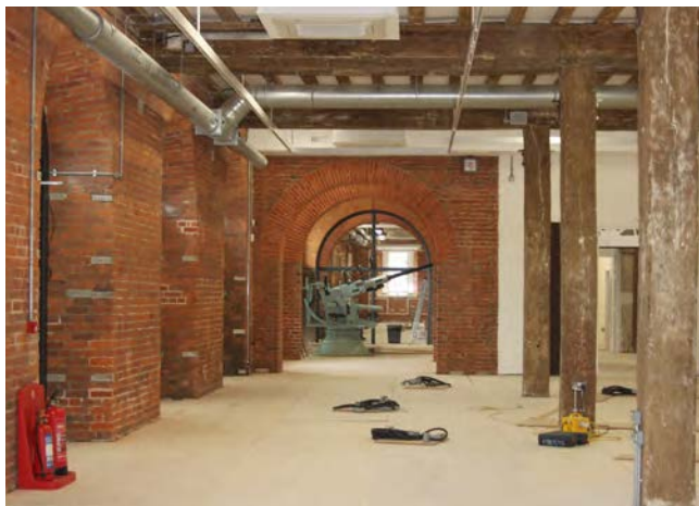
Above: Fig. 312. Ground floor of Portsmouth Storehouse No. 10 (1776, 1/59) looking south along the eastern bay, showing renewed brickwork and timber pillars and beams during its refurbishment for the twentieth century Babcock Galleries (2014) A. Coats 2013. Reproduced by kind permission of the Trustees of the National Museum of the Royal Navy.
