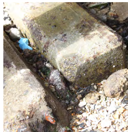
Fig. 237. Unused reinforced concrete beams lying beneath Portsmouth Boathouse No. 4 (1940, 1/6). A. Coats 2015. Reproduced with the kind permission of Portsmouth Naval Base Property Trust.
