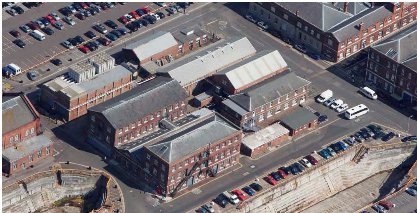
Fig. 372. 23852/27 SU 6300/81. Aerial photograph of the Block Mills from the southwest, before its refurbishment in 2007-8, when the external staircases were removed (11 Apr 2005). ©Historic England.
