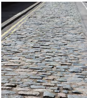
Fig. 330. In Portsmouth Admiral's Walk, a seven foot wide section of setts running along the north side of 1/81 (c.1850–90). A. Coats 2013. Reproduced with the permission of the MoD.
