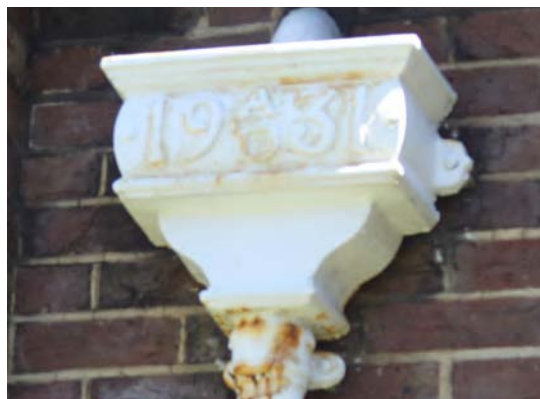
Fig. 331. Rainwater hopper dated 1931 on Portsmouth South Office Block Annexe (1931, 1/87C). A. Coats 2013. Reproduced with the permission of the MoD.
