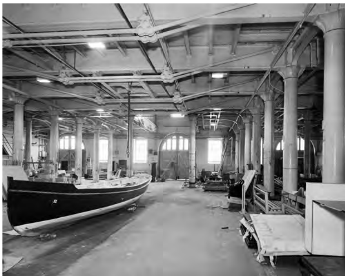
Fig. 261. BB012875. Photograph of the ground floor interior of Portsmouth Boathouse No. 6 from the northeast, before refurbishment in 2001 (11 Jun 1991). ©Crown copyright.HE.
