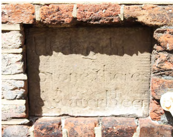
Fig. 199. Set into the south elevation of Portsmouth Building 1/81 is a dressed Portland stone or replacement concrete plaque which reads 'Under this Stone there is a water Beer', marking an old well or water tank surviving from the seventeenth century dockyard. This would have supplied the garden to the original Commissioner's House (1666) which lay north of Stony Lane until the house was demolished in the 1780s. A. Coats 2013. Reproduced with the permission of the MoD.
