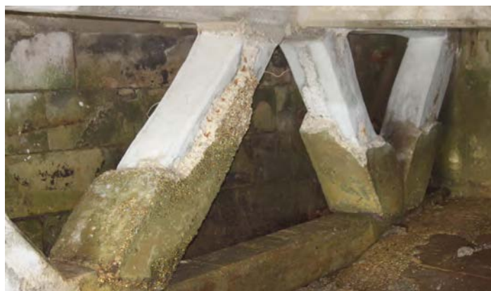
Fig. 234. Northern extent (east end) of the concrete and steel trusses forming the undercroft of Portsmouth Boathouse No. 4 (1940, 1/6) showing the eighteenth century Portland stone north seawall and slipway stones. Concrete repairs to the trusses were carried out in 2014–15. A. Coats 2015. Reproduced with the kind permission of Portsmouth Naval Base Property Trust.
