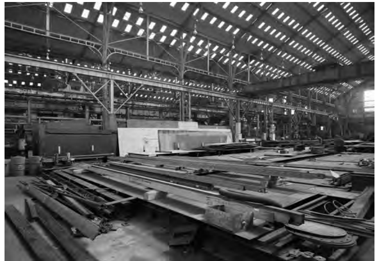
Fig. 369. J297/11. Photograph of the interior of Ship Shop Nos 3-4 before their demolition in 1980 (23 June 1971). ©Crown copyright.HE.
