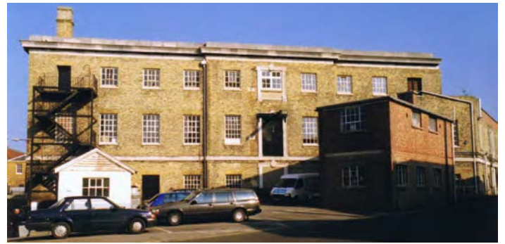
Fig. 265. Portsmouth Boathouse No. 6. Photograph of the south elevation. PNBPT Record Photograph no. E02 (June 1998). Reproduced with the kind permission of Portsmouth Naval Base Property Trust.
