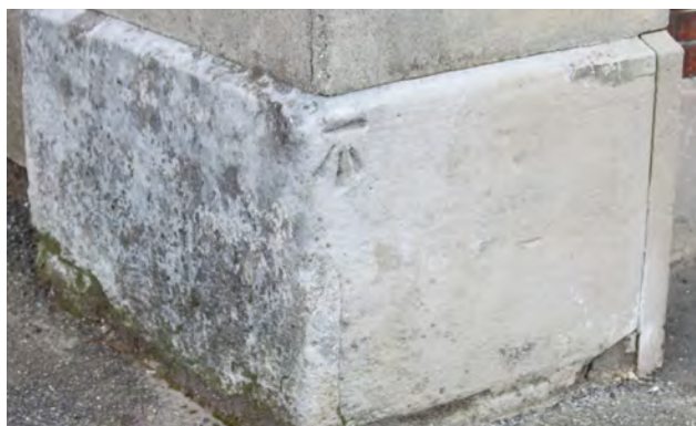
Fig. 355. Plinth bearing a broad arrow at the base of the western gate pier of the first Portsmouth Marlborough Gate (1711, 1/138). A. Coats 2013. Reproduced with the permission of the MoD.
