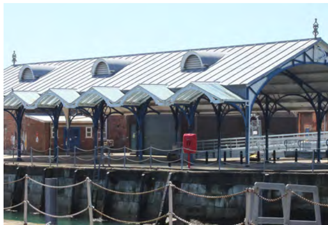
Fig. 295. Portsmouth Railway Shelter (1893, 1/45) on South Railway Jetty, re-sited since c.2000 on the west quay of the North Camber. A. Coats 2013. Reproduced with the permission of the MoD.
