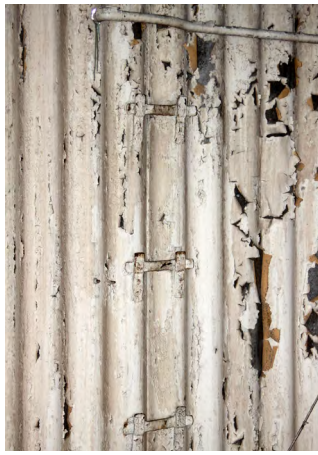
Fig. 327. Original corrugated iron and fittings inside Portsmouth Fire Station (1843, 1/77). A. Coats 2012. Reproduced with the permission of the MoD.
