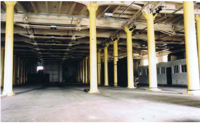
Fig. 264. Portsmouth Boathouse No. 6. Photograph of the ground floor, looking east showing the cast iron pillars and trusses. PNBPT Record Photograph no. G41 (June 1998). Reproduced with the kind permission of Portsmouth Naval Base Property Trust.
