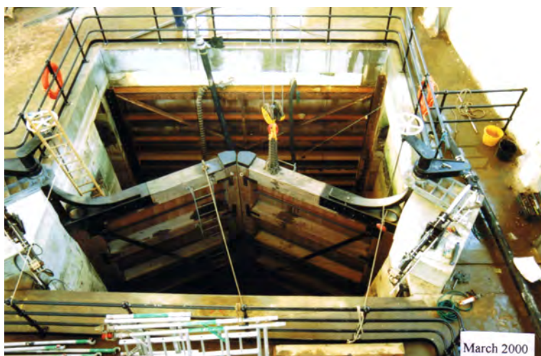
Fig. 249. Photograph of Portsmouth Boathouse No. 4 lock gates: adjustments to gates (PNBPT, 1.3.2000 no. 53). Reproduced with the kind permission of Portsmouth Naval Base Property Trust.
