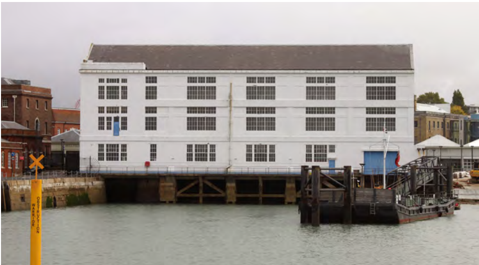
Fig. 230. West (harbour) elevation of Portsmouth Boathouse No. 4 (1940, 1/6). A. Coats 2015. Reproduced with the kind permission of Portsmouth Naval Base Property Trust.
