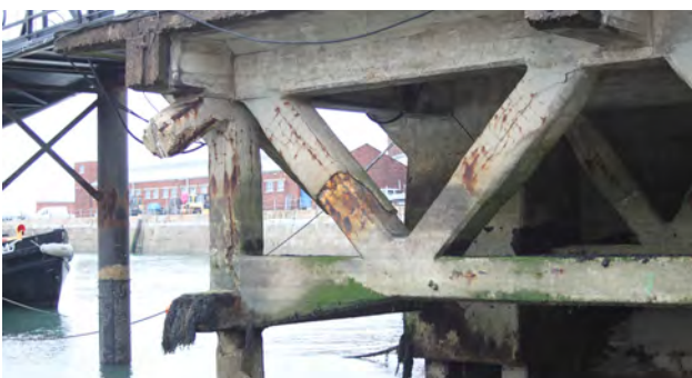
Fig. 231. Southern extent of the concrete and steel trusses forming the undercroft of Portsmouth Boathouse No. 4 (1940, 1/6) on its west (harbour) elevation. A. Coats 2015. Reproduced with the kind permission of Portsmouth Naval Base Property Trust.
