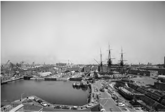
Fig. 334. J195/01/71. Photograph of Basin No. 1 and Docks 1-5 looking east pre- Mary Rose and pre-Monitor HMS M33 (28 Apr 1971). ©Crown copyright.HE.
