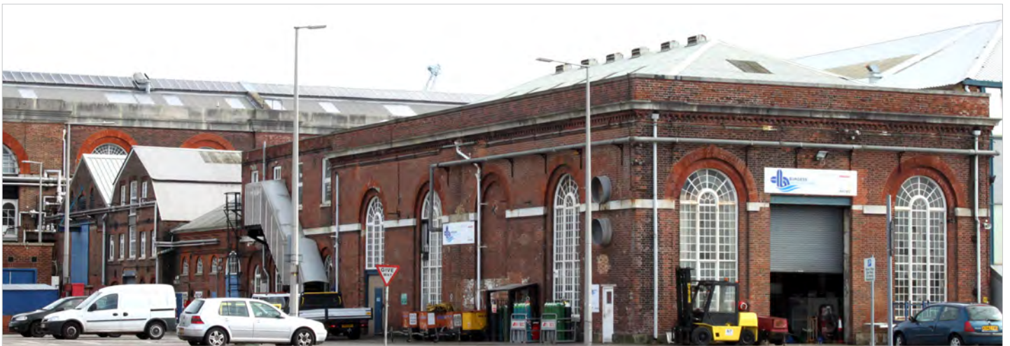
Fig. 379. Former 80hp Portsmouth Engine House (1849, 1/209) from the northeast, with the Steam Factory in the background. A. Coats 2014. Reproduced with the permission of the MoD.
