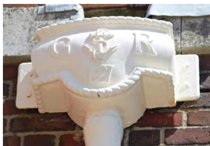
Fig. 298. Rainwater hopper dated 1927, Portsmouth Victory Gallery (1938, 1/57, NMRNP). A. Coats 2013. Reproduced by kind permission of the Trustees of the National Museum of the Royal Navy.
