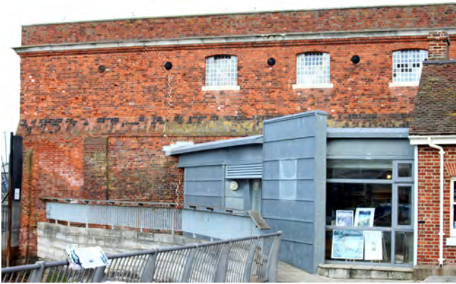
Fig. 211. Former Portsmouth Naval Recruiting Office (1862, 1/1, PNBPT) with the additional wing created by Portsmouth City Council for use as a Tourist Information Centre (2001). A. Coats 2013. Reproduced with the kind permission of Portsmouth Naval Base Property Trust.
