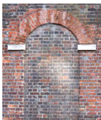
Fig. 208. Blocked gateway through the Dockyard Wall at Bonfire Corner which was aligned with the first (1704–c.1784) Dockyard Chapel. A. Coats 2012. Reproduced with the permission of the MoD.
