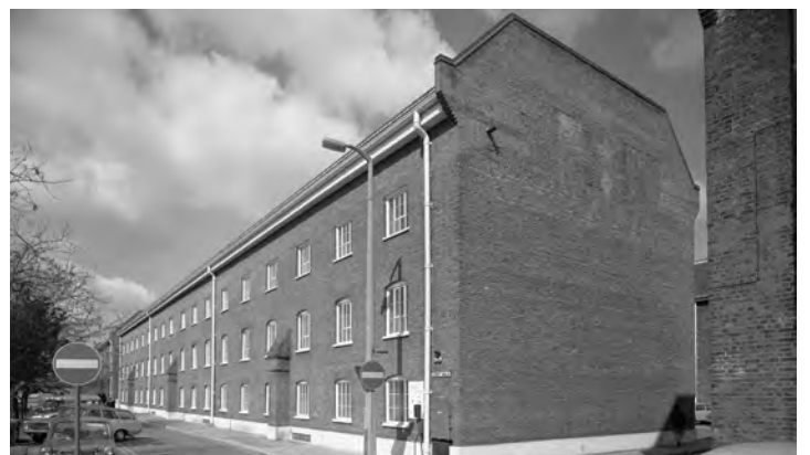
Fig. 318. J188/03/71. Photograph of Storehouse Nos 15, 16 and 17 (28 Apr 1971) from the east, showing 'GR 1771' inserted in darker bricks on the east elevation of Storehouse No. 16. ©Crown copyright.HE.
