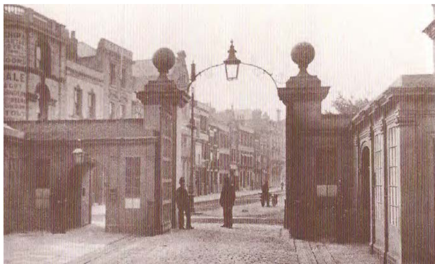
Fig. 204. Photograph of the north elevation of the Main (now Victory) Gate in 1895, showing its original width. Courtesy of Portsmouth Royal Dockyard Historical Trust.
