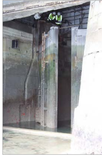
Fig. 240. Lock entrance to Portsmouth Boathouse No. 4 (1940, 1/6), showing the wooden lock gates which connect the channel running beneath Boathouse No. 4 and into the Mast Pond with the harbour. On the right is the battered eighteenth century Portland Stone sea wall, at the top a reinforced concrete beam supporting the building, and on the left shuttered concrete above Portland stone. A. Coats 2015. Reproduced with the kind permission of Portsmouth Naval Base Property Trust.
