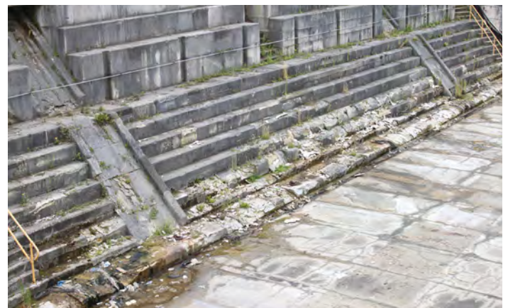
Fig. 339. Portsmouth Dock No. 6 (1700), showing disintegration of the lower altar stones through weathering. Following the straightening of the western jetties for the new Queen Elizabeth class aircraft carriers in the early 2000s, it is no longer connected to the harbour and no longer has the environmental protection of seawater. A. Coats 2012. Reproduced with the permission of the MoD.
