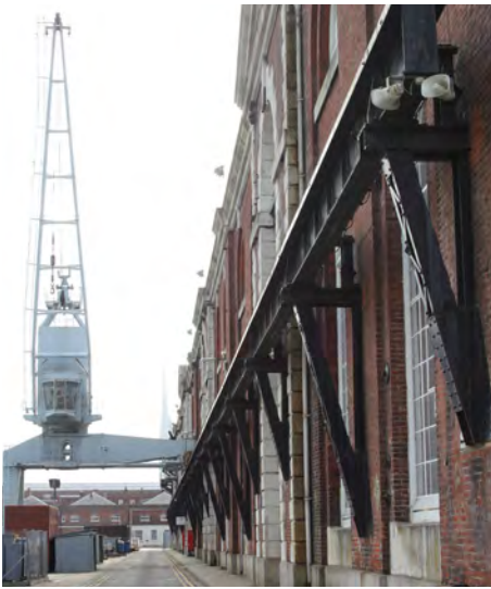
Fig. 376. Portsmouth Steam Factory (1847, 1/208), east elevation, showing the 10 ton gantry crane. A. Coats 2013. Reproduced with the permission of the MoD.
