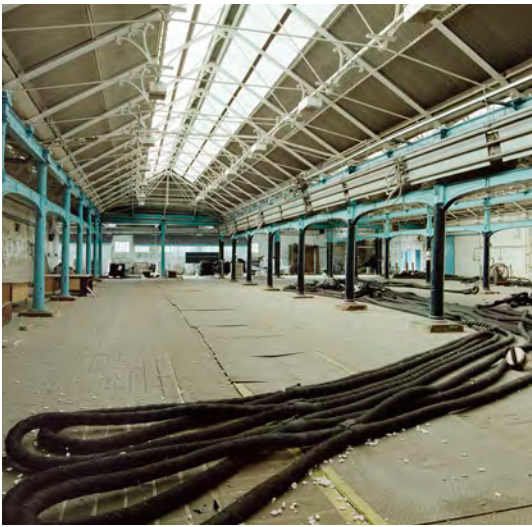
Fig. 291. AA045925. Photograph of the interior of the Chain Test House looking south. (9.7.2003). ©Historic England.
