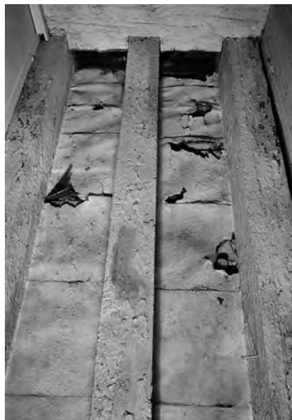
Fig. 310. J360/06/72. Photograph of Storehouse Nos 9, 10, 11: Mr Hartley's fire plates on first floor joists and floorboards (c.1971). ©Crown copyright.HE.
