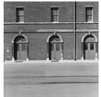
Fig. 311. AA98/04650. Portsmouth Dockyard prints FL00981. Photograph by Eric de Mare of the eastern elevation of Portsmouth Storehouse No. 10, with the railway track in evidence. (1956). The doorways were modified for the NMRN twentieth century Babcock Galleries (2014). Reproduced by permission of Historic England.
