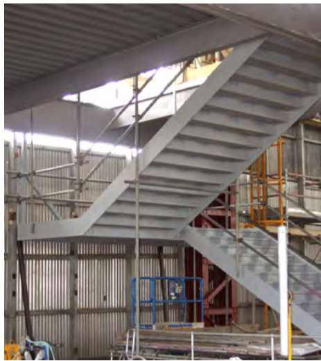
Fig. 242. Interior of the corrugated steel wall forming the south elevation of Portsmouth Boathouse No. 4 (1940, 1/6), showing the newly constructed stairway and mezzanine floor. A. Coats 2015. Reproduced with the kind permission of Portsmouth Naval Base Property Trust.
