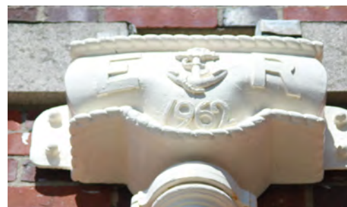
Fig. 300. Rainwater hopper dated 1962, Portsmouth Victory Gallery (NMRNP, 1938, 1/57). A. Coats 2013. Reproduced by kind permission of the Trustees of the National Museum of the Royal Navy.
