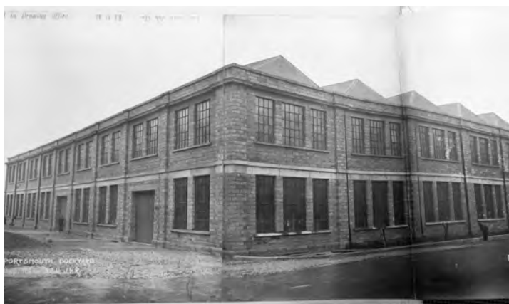
Fig. 340. Portsmouth Joiners Shop 3.2.1911. TNA, ADM 195/79 (1857–1915). 100 photographs depicting: construction works at Portsmouth Dockyard. Reproduced with the permission of The National Archives.
