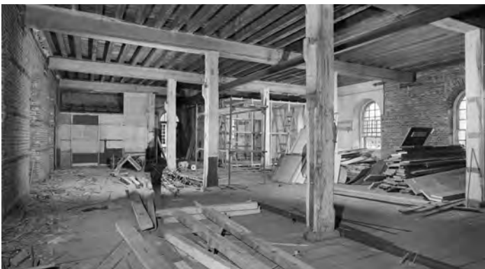
Fig. 307. J106/04/72. Photograph of Storehouse No. 11, ground floor conversion to the McCarthy Museum (28 Apr 1971). ©Crown copyright.HE.
