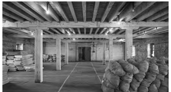
Fig. 308. J186/05/71. Photograph of Storehouse Nos 9, 10 or 11 (28 Apr 1971). ©Crown copyright.HE. It is hoped that the particular storehouse can be identified.
