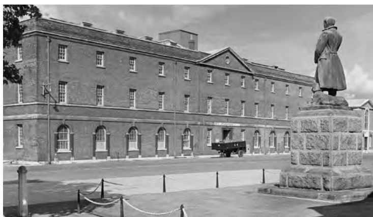
Fig. 303. AA98/04645. Portsmouth Dockyard prints FL00981. Photograph of the eastern elevation of Portsmouth Storehouse No. 11 taken from outside South Office Block Annexe (1931, 1/87C) by Eric de Mare (1956). The statue of Captain Robert Falcon Scott was in this spot following the Second World War until 2000, when it was moved to the Porter's Garden. Reproduced by permission of Historic England.
