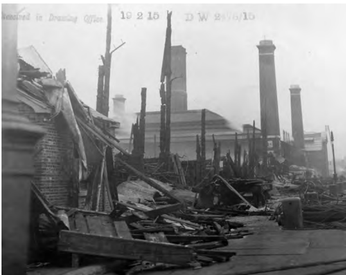
Fig. 360. Damage to Portsmouth No. 1 Slip Jetty looking east, 1.2.1915, with the Smithery and the Steam Factory in the background. TNA, ADM 195/79 (1857–1915). 100 photographs depicting: construction works at Portsmouth Dockyard. Reproduced with the permission of The National Archives.
