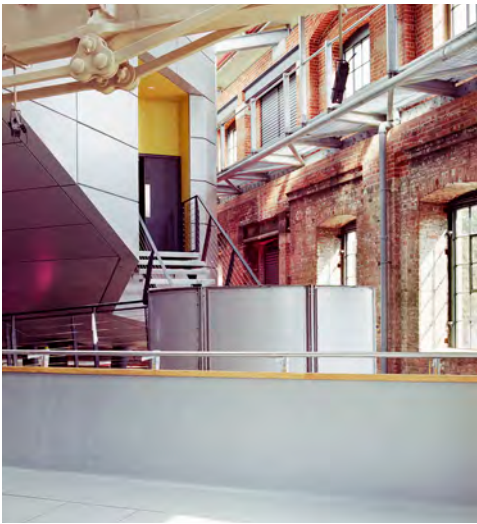
Fig. 275. AA026355. Photograph of the eastern interior of Portsmouth Boathouse No. 6 showing the cinema structure inserted within the area damaged by a bomb in the Second World War (2001). ©Historic England.
