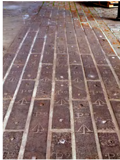
Fig. 292. AA045923. Photograph of the floor of the Chain Test House, the pathway consisting of Portsmouth Dockyard cast iron ballast pigs (9.7.2003). ©Historic England.
