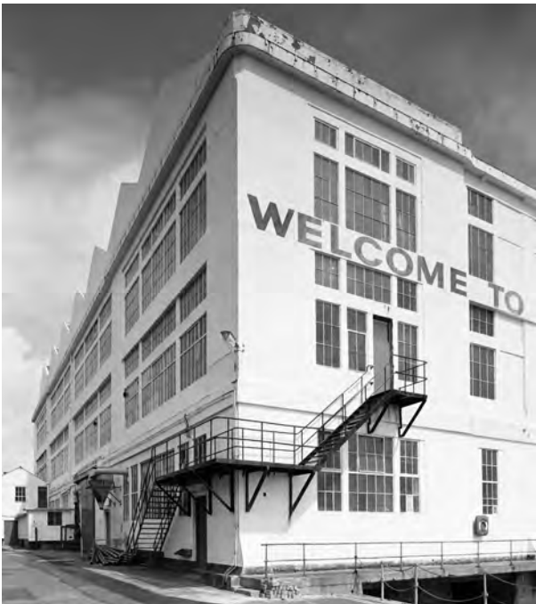
Fig. 228. BB97/09275. Photograph of Portsmouth Boathouse No. 4 from the north west corner (28 July 1997). ©Crown copyright.HE.
