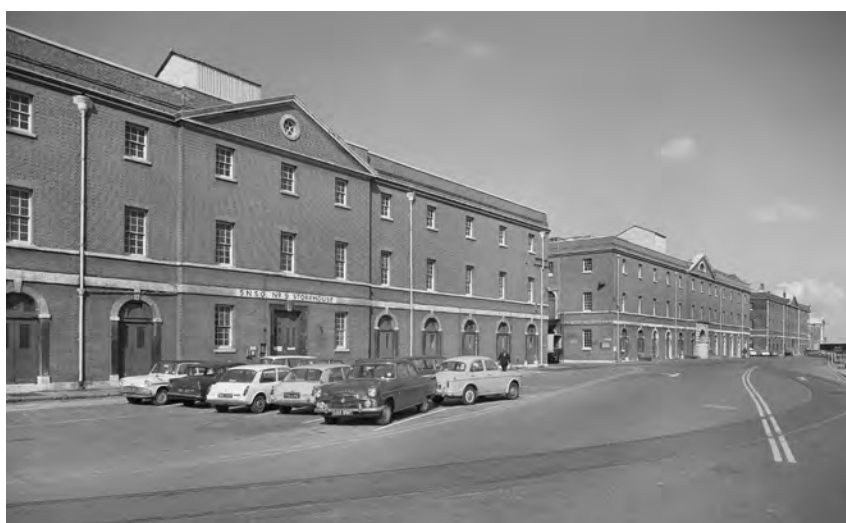
Fig. 302. J186/01/71. Photograph of the west elevations of Storehouse Nos 9, 10 and 11 (28 Apr 1971). ©Crown copyright.HE.
