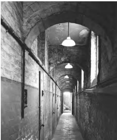
Fig. 214. J473/03/71. Photograph of the Cell Block Interior: ground floor looking east/west (8 Oct 1971). ©Crown copyright.HE.
