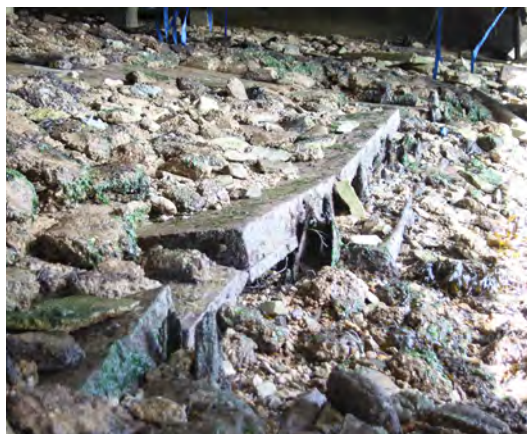
Fig. 235. Lowest level of the eighteenth century Portland Stone slipway stones, held in place by a line of wooden posts, visible beneath a layer of solidified bags of concrete, below Portsmouth Boathouse No. 4 (1940, 1/6). A. Coats 2015. Reproduced with the kind permission of Portsmouth Naval Base Property Trust.
