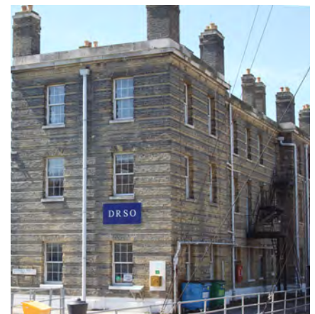
Fig. 296. Former Office for the Portsmouth Captain of the Yard/Harbour Master (c.1850, 1/53), now the Disposal & Reserve Ships Organisation. A. Coats 2013. Reproduced with the permission of the MoD.
