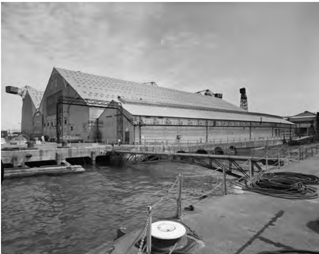
Fig. 368. J297/06. Photograph of Ship Shop Nos 3-4, south of Slip No. 5, before their demolition in 1980 (23 June 1971). ©Crown copyright.HE.
