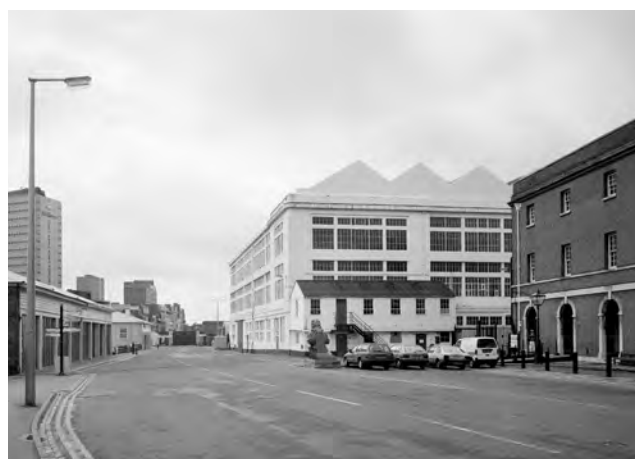
Fig. 250. BB97/012856. Photograph of the northwest corner of Portsmouth Boathouse No. 4 with Boathouse No. 4 Annex on the north side (28 Jul 1997). ©Crown copyright.HE.
