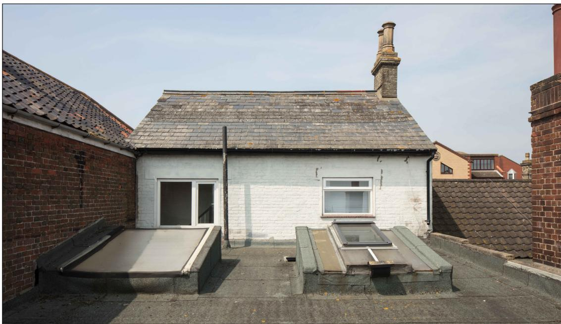
*Fig 13 The flat roof of the rear wing looking west, showing the faint scar of the original roof. (Historic England, Patricia Payne, DP232175)*
