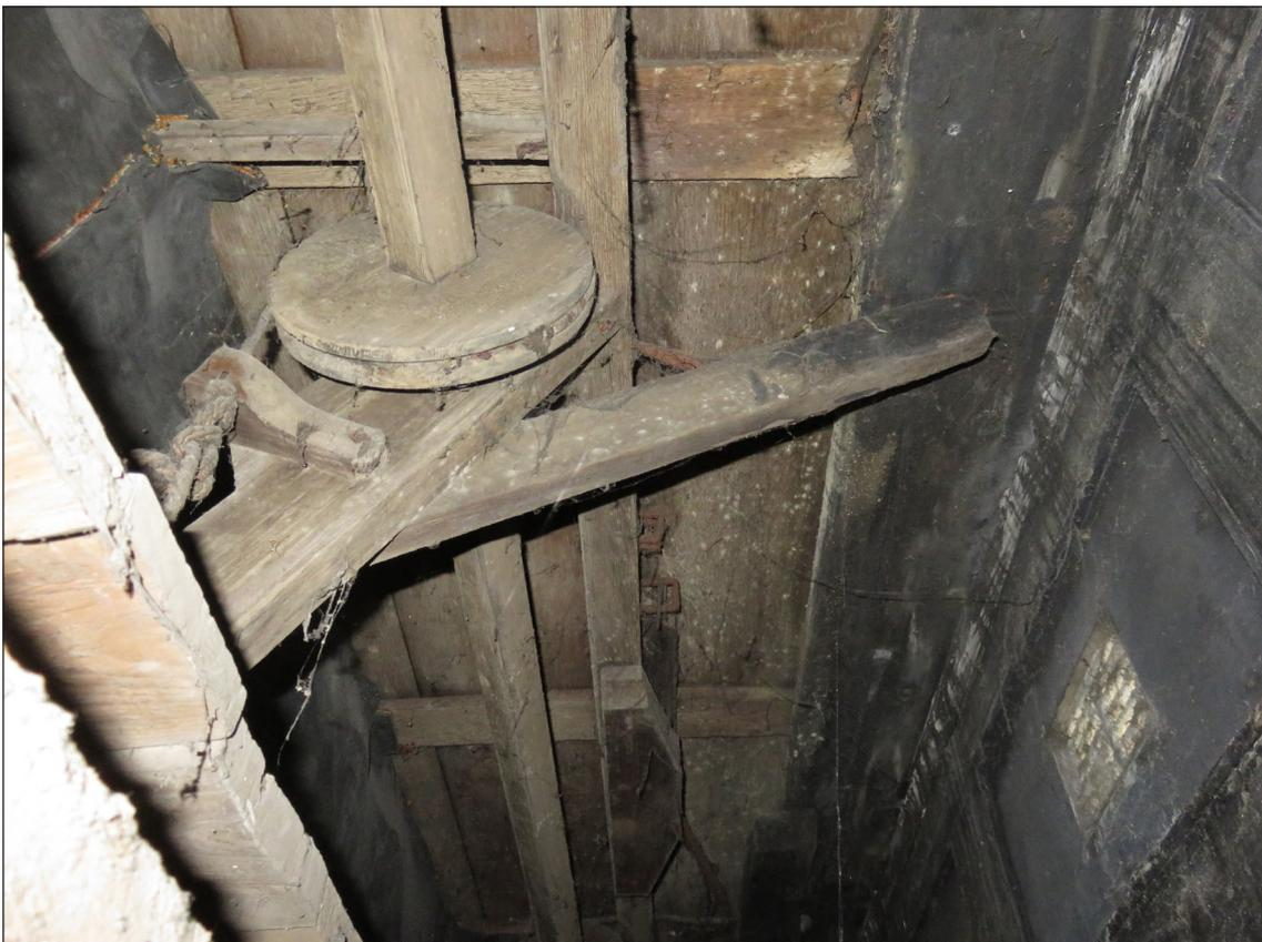
*Fig 26 Detail of mechanism for operating shop shutters, looking up into space under stall board. (Historic England, K. Morrison)*
