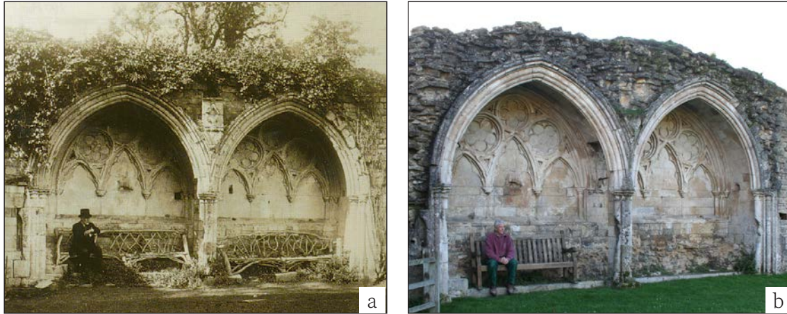
Figure 7.2 (a) The Kirkham Priory laver site in the 19th century, covered with extensive natural vegetation growth and (b) in recent times, where past conservation techniques have led to the removal of the protective vegetation cover (© Chris Wood, Historic England ).
