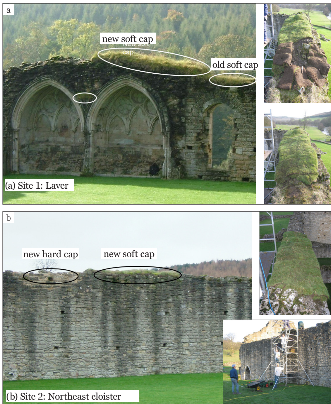
Figure 2.5 Location of newly installed soft capping at Kirkham Priory. (a) Site 1, the laver alcove, where a 5 m long (1.3 m wide) section of 10 cm thick soft capping (using local turf and soil containing regolith) was installed on the top of the wall (see insets of installation). A 30-cm (15-cm wide) section was also installed, at the top of the column between the arches (lower white circle). (b) Soft capping (3.9 m long, 50 cm wide 10 cm thick soft capping using local turf and soil with regolith) and hard capping (3.9 m, 50 cm wide using lime mortar and stone) on the north east cloister wall, at site 2. (all ©Heather Viles, University of Oxford)
