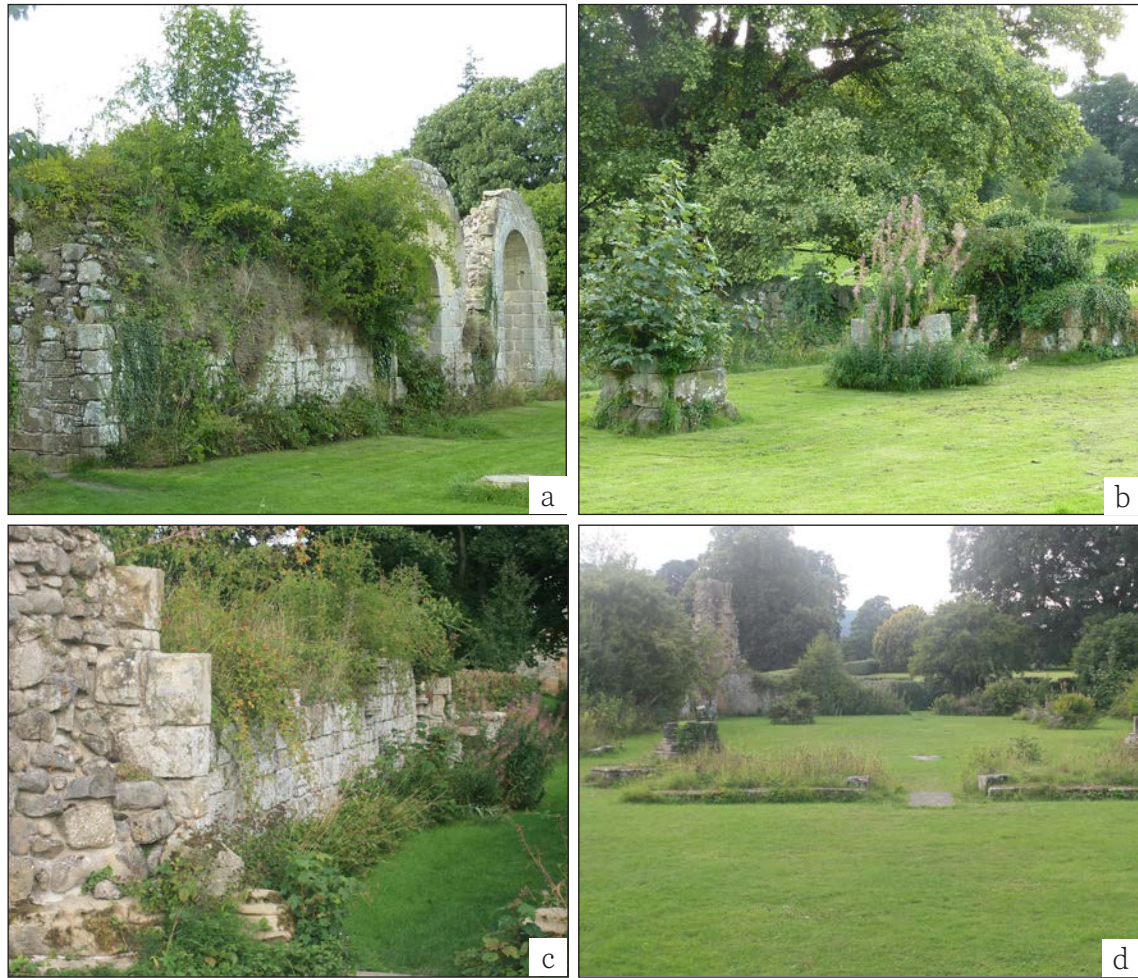
Figure 1.4 (a-d) Natural soft capping and deliberate planting at Jervaulx Abbey. (a,c Chris Wood ©Historic England; b, d ©Heather Viles University of Oxford)
