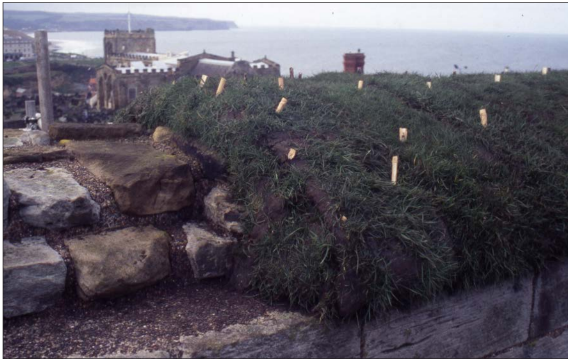
Figure 6.4 When capping steeply profiled edges it is critical to peg the turf in place until it can properly root into the mass of soil beneath. ©Alan Cathersides
