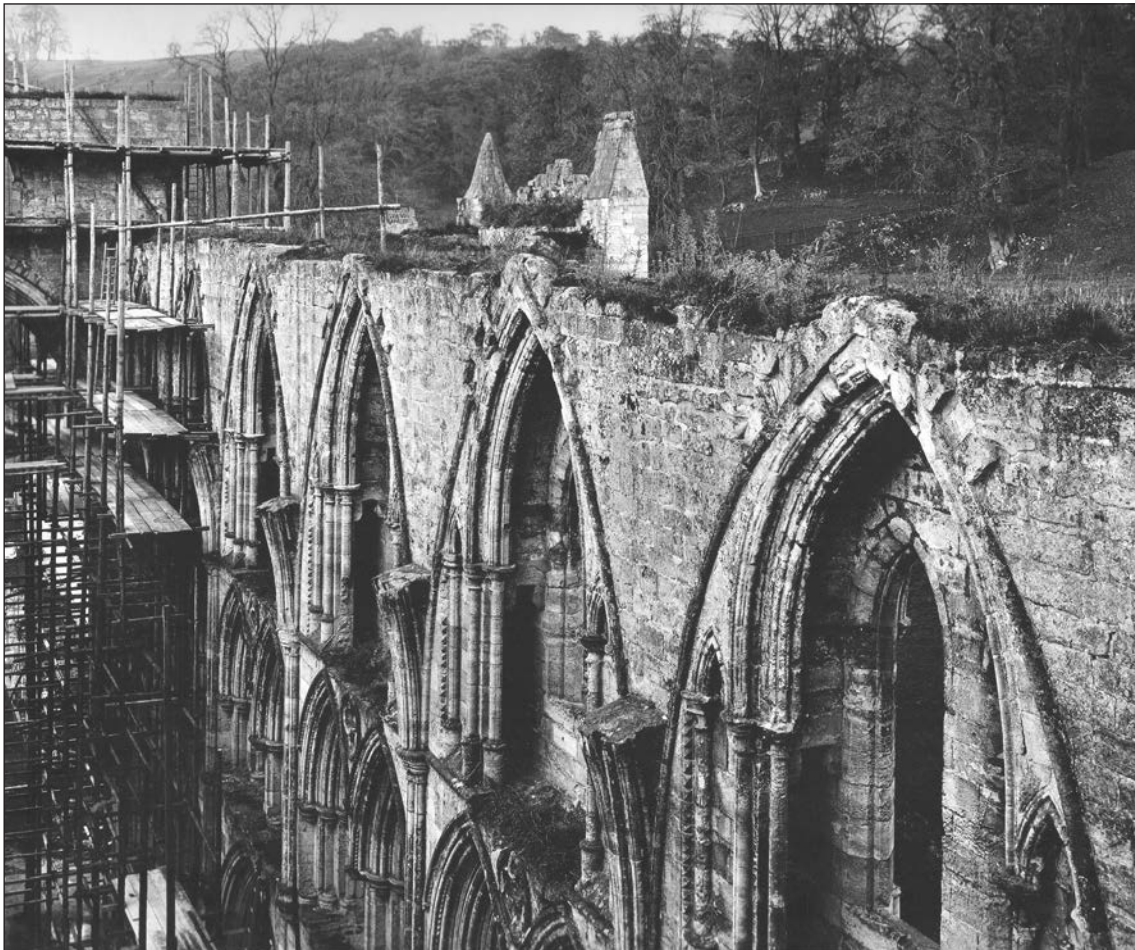
Figure 7.1 An early photograph showing the Church at Rievaulx before the Ministry of Works began consolidation in the early 20th Century. A natural soft capping had developed over the previous 350 years and seems to have provided good protection for the masonry below. Source: Historic England Archive (AL0876_011_01)
