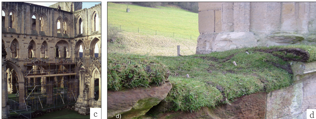
Figure 2.8 c, d The soft capping installed high at triforium level in the wall of the main abbey church nave at Rievaulx. (both ©Heather Viles, University of Oxford)
