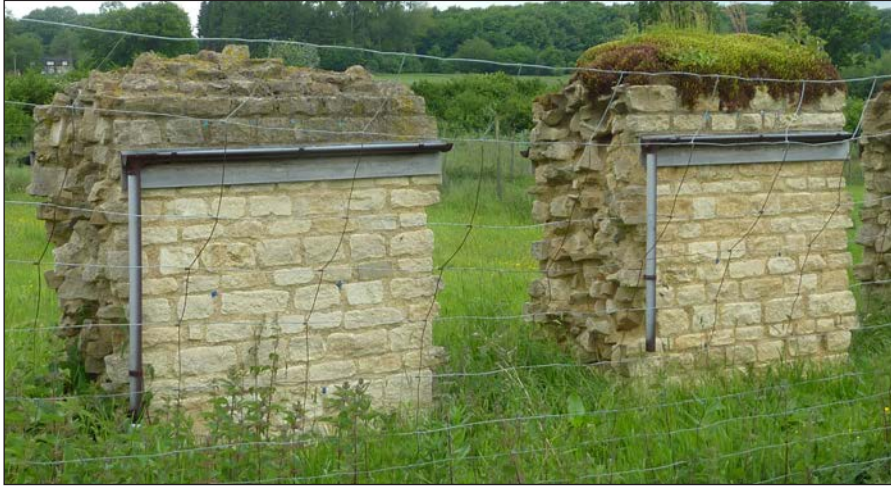
Figure 4.27 Dark colouration on the top two courses of stonework on hard-capped but not on the soft-capped walls at Wytham Woods.
