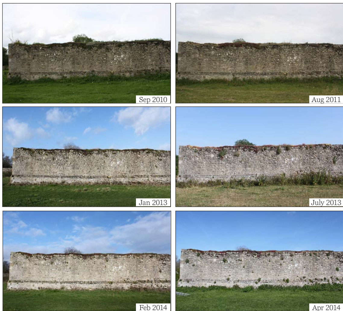
Figure 4.37 Changes in appearance to grass and sedum soft capping at Godstow Nunnery. ©Heather Viles, University of Oxford
