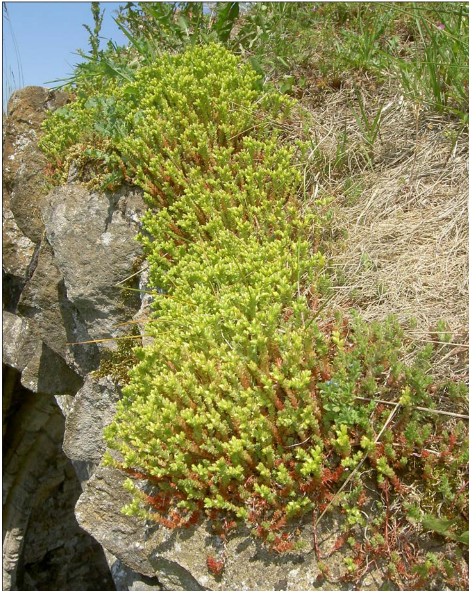
Figure 5.1 Naturally occurring sedums forming stable edges on older soft caps at Kirkham Priory. ©Alan Cathersides
