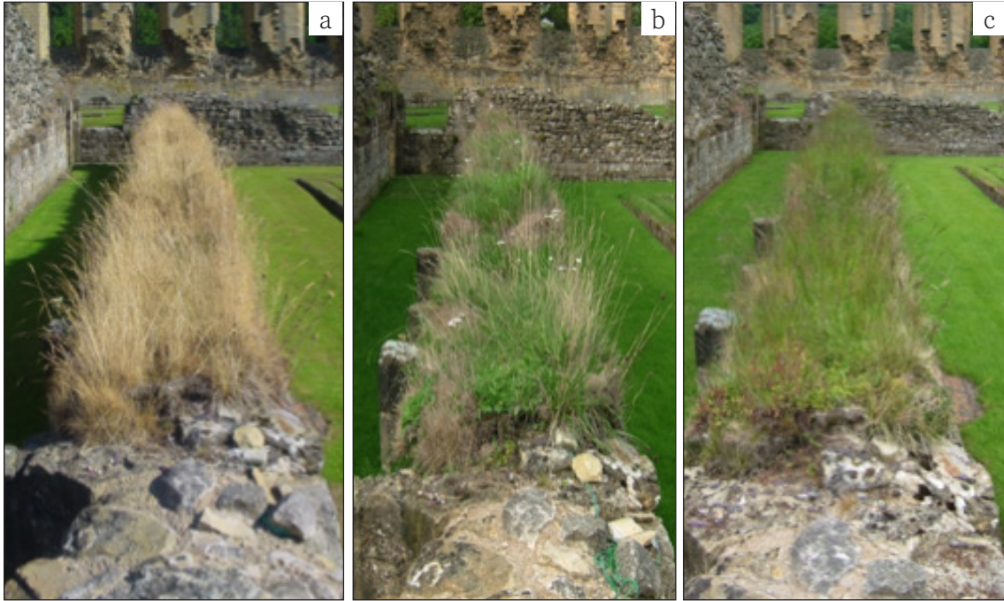
Figure 6.9 A soft-capped section, at Byland Abbey completely dried out in August 2006 (a), greening up a few weeks later in September 2006 (b) and completely recovered by June 2007 (c). (all ©Heather Viles, University of Oxford)
