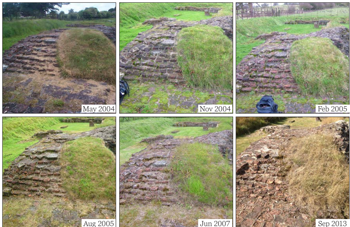
Figure 4.33 Changing appearance of soft capping at Thornton Abbey. ©Heather Viles, University of Oxford
