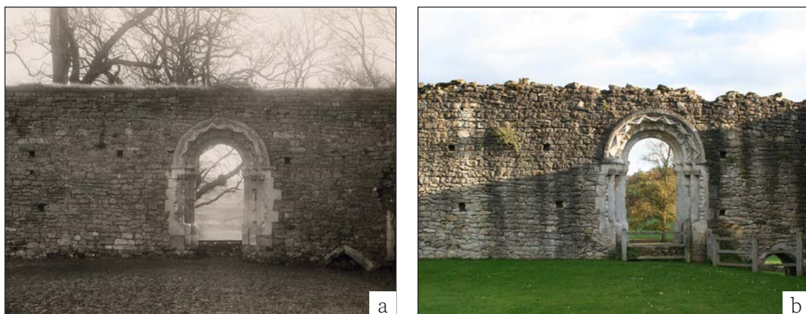
Figure 7.3 (a) Kirkham Priory refectory wall in the early 20th century before consolidation, showing clear coursing lines of the facework and a very flat walltop with a grass cover, and (b) in recent times, without a grass cover and significant alterations to its profile (© Chris Wood, Historic England ).
