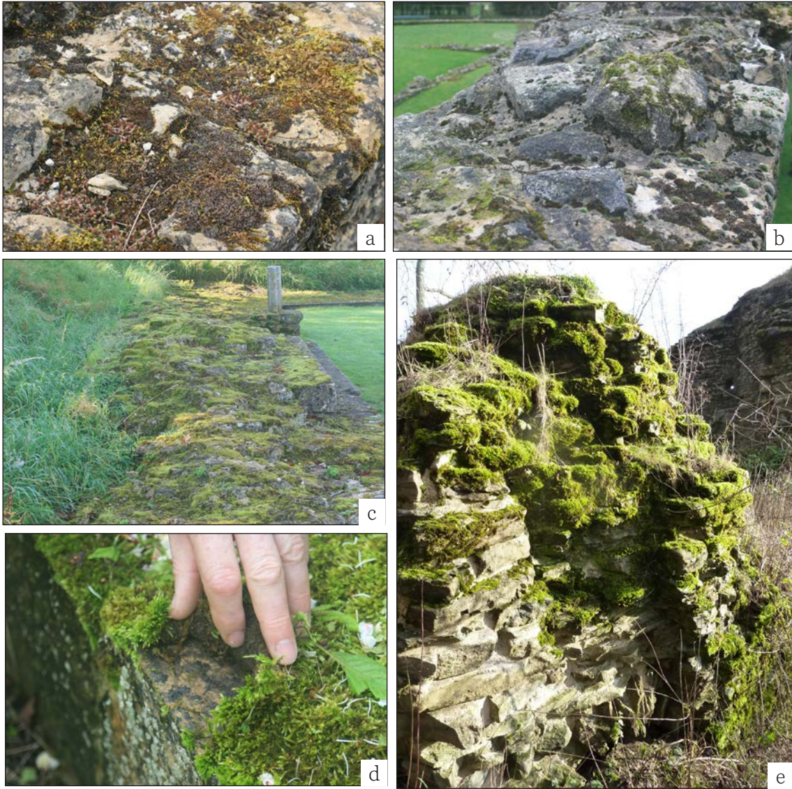
Figure 1.12 Natural growth of lichens and mosses on wall heads. (a-b) Kirkham Priory, (c-d) Hailes Abbey and (e) Wigmore Castle. (a-d) © Alan Cathersides, (e) Chris Wood ©Historic England)
