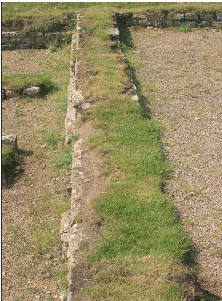
Figure 6.9 A soft-capped section, at Byland Abbey completely dried out in August 2006 (a), greening up a few weeks later in September 2006 (b) and completely recovered by June 2007 (c). (all ©Heather Viles, University of Oxford)
