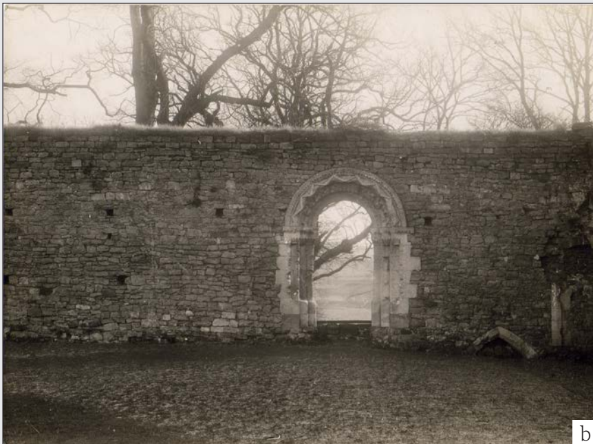
Figure 1.15 (a) Natural capping at Rievaulx, (b) Natural capping at Kirkham reredorter.
