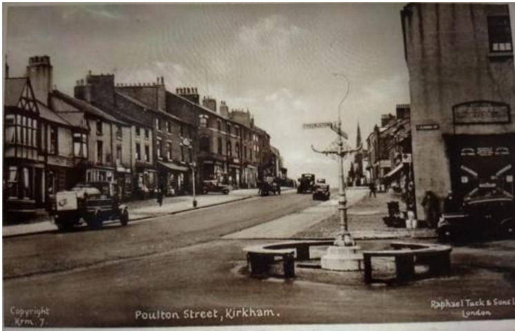
Figure 6. Poulton Street, Kirkham, Lancashire © Helen Shearn Associates
