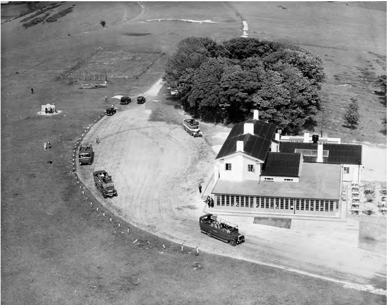
Figure 67: Aerial view of the Dyke Hotel with the commemorative seat visible to the left. Note the four visitor motor buses and three cars in the hotel car park. EPW041379 01-MAY-1933 © Historic England Archive. Aerofilms Collection.
