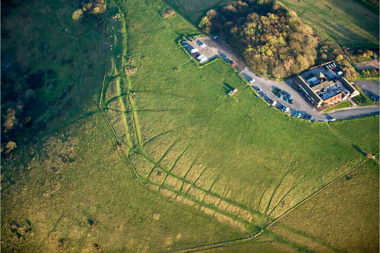
Figure 68: View of the current Dyke Hotel and part of the ramparts of the hillfort cut by numerous paths and commemorative bench in the foreground. The former funicular foundation cutting can be seen in the shadowed area top left. 24801_011 29-OCT-2007 © Historic England Archive.
