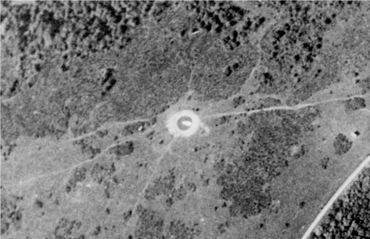
Figure 37: A dewpond near Highpark Corner photographed in 1928. This has largely been levelled but the lidar shows it survives as a slight depression. Detail of Historic England Archive CCC 8848/2952 11-JUL-1928. © Historic England Archive. Crawford Collection.
