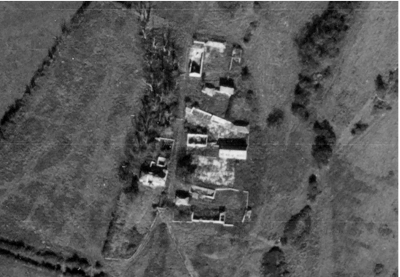
Figure 26: The damaged and roofless buildings of Balmer Farm because of Second World War army training exercises. Detail of RAF/CPE/UK/1768 RS 4218 7-OCT-1946 Historic England Archive (RAF Photography).
