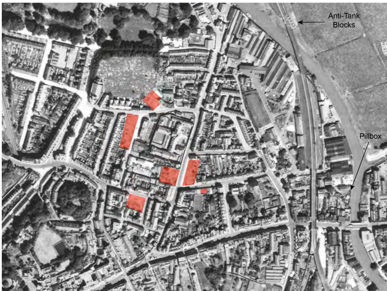
Figure 85: Bomb damage in the centre of Lewes (highlighted in red). Note the anti-tank blocks to prevent the enemy from crossing the river via the railway bridge. The main road bridge across the river (bottom right) was wired with explosives. Detail of RAF/106G/UK/538 RP 3120 24-JUL-1945 Historic England Archive (RAF Photography).
